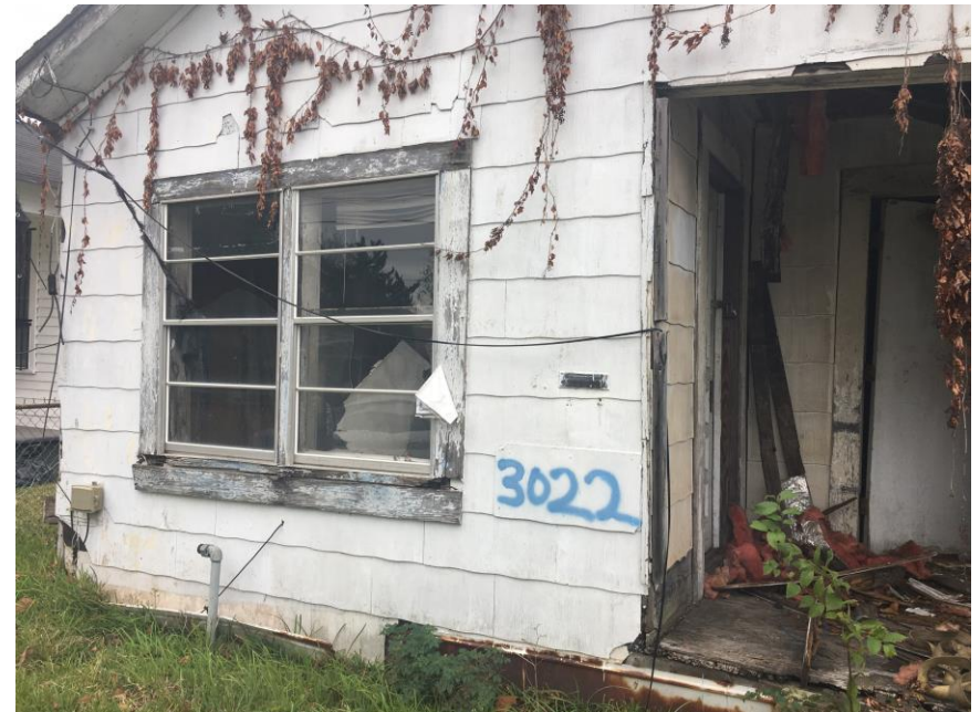
Photograph No. 4 View of HA-04: White Cementous Panels (Transite)
