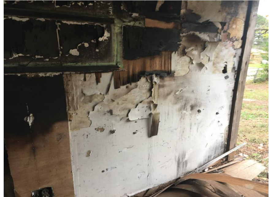
Photograph No. 2 View of HA-02: White Sheetrock
