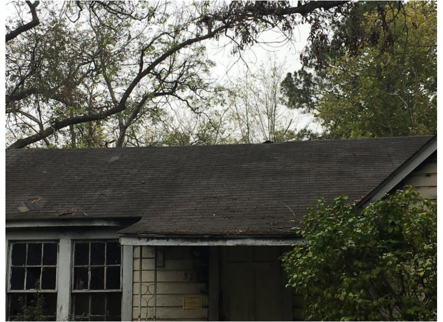
Photograph No. 6 View of HA-06: Black Roof Shingle with Felt Paper
