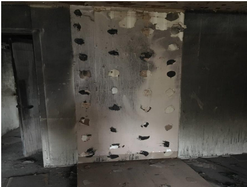
Photograph No. 3 View of HA-03: Black Wall Panel Glue Dot with White Texture
