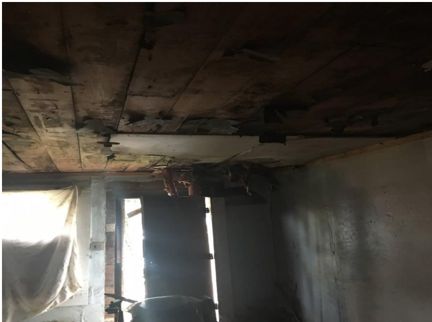
Photograph No. 3 View of HA-03: White Sheetrock, Tape & Mud-Ceiling
