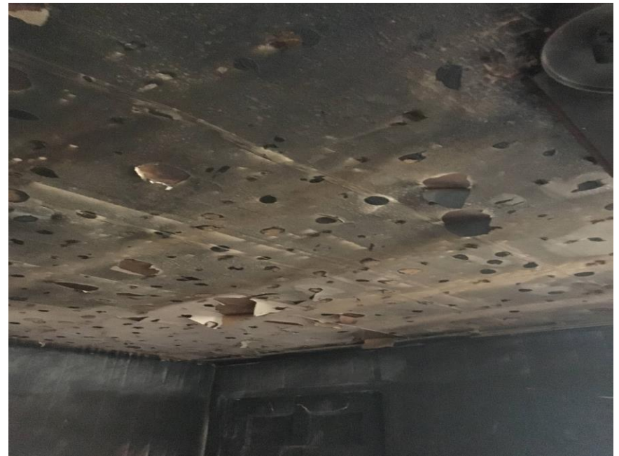
Photograph No. 4 View of HA-04: Black Ceiling Tile Glue Dot with White Texture
