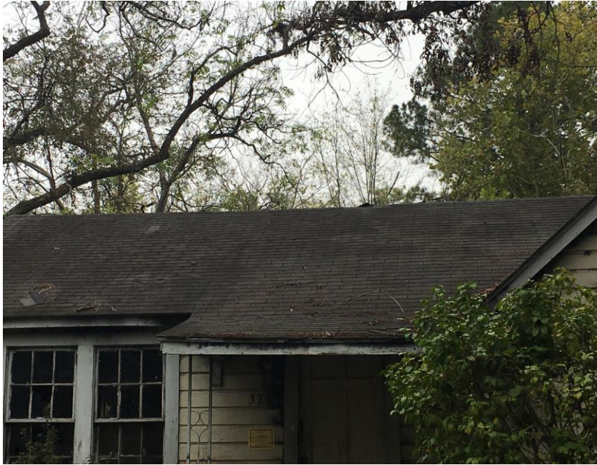
Photograph No. 5 View of HA-05: Window Pane Glazing
