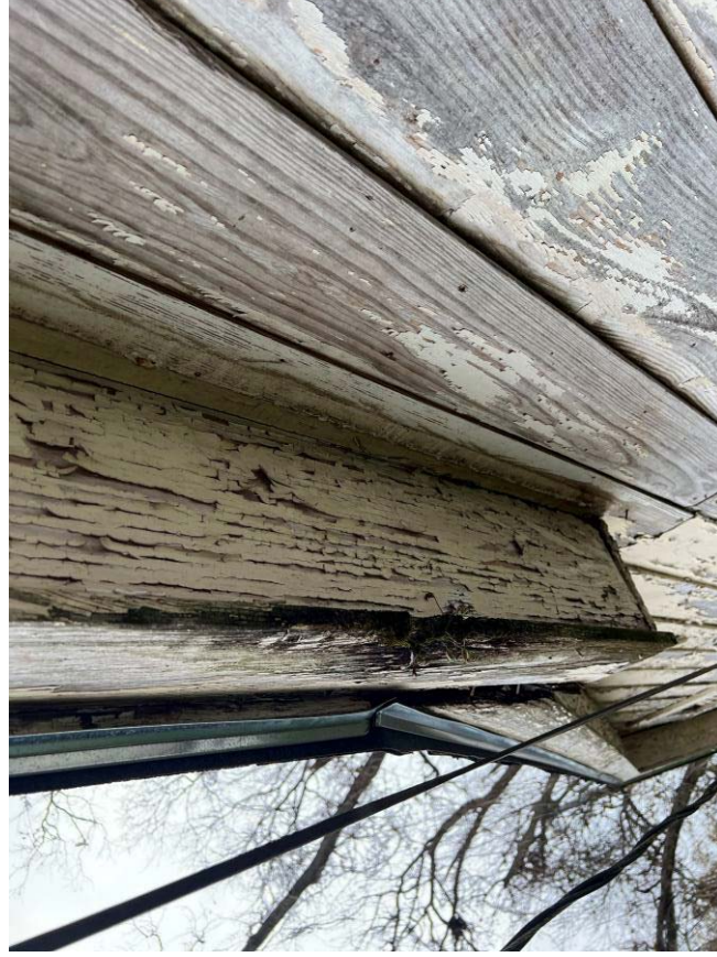
View of deteriorated LBP at Exterior Wall B – Roof Deck (Soffit)
