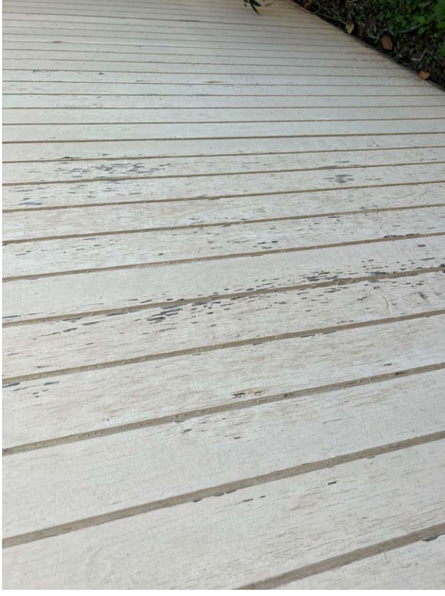
View of deteriorated LBP at Exterior Wall D - Wall
