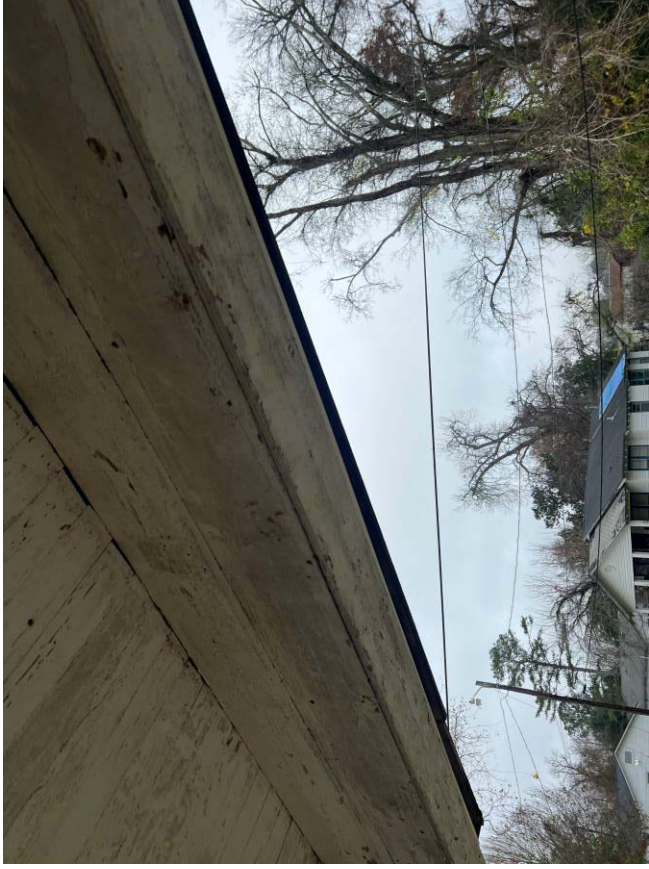
View of deteriorated LBP at Exterior Wall A - wall cap.
