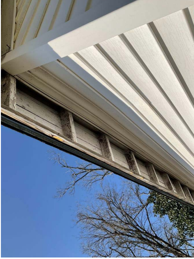
View of deteriorated LBP at Exterior Wall B - rafter tails.
