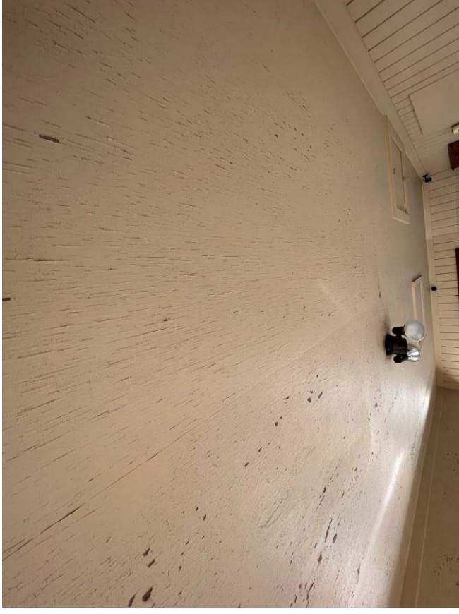
View of deteriorated LBP at Carport - Ceiling
