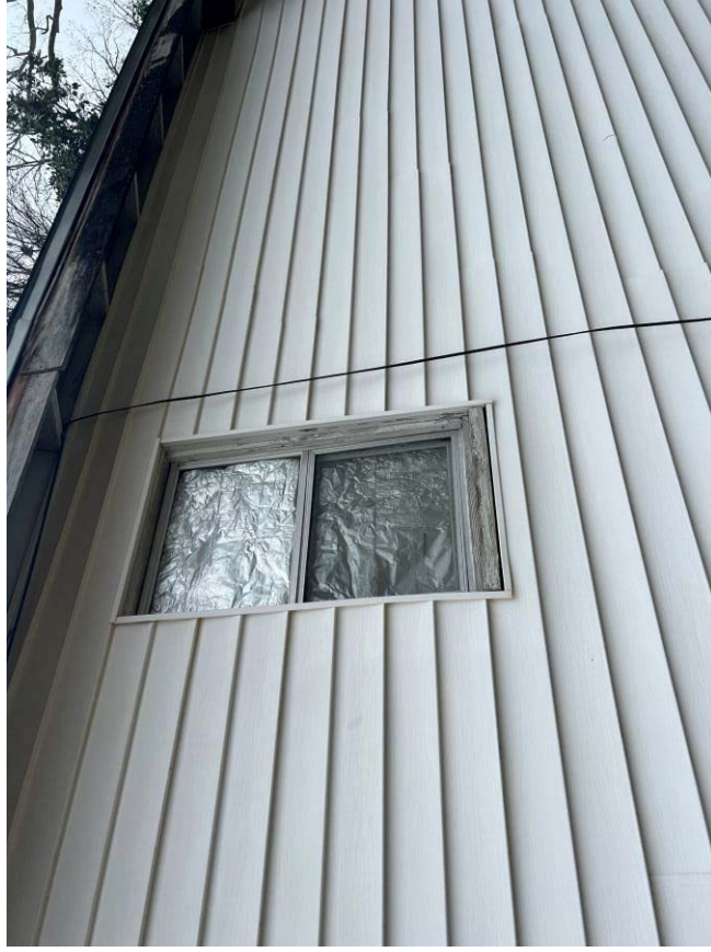
View of deteriorated LBP at Exterior Wall D - Window 11
