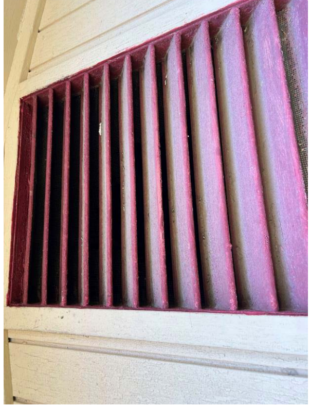
View of deteriorated LBP at Exterior Wall D - Gable Vent
