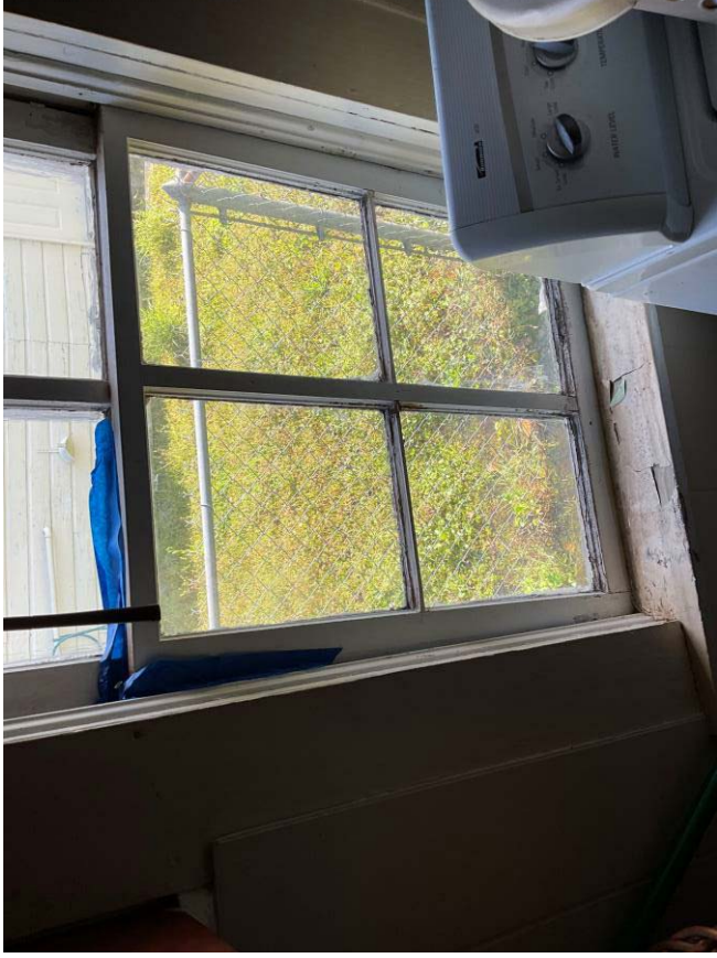
View of Window 5 – Deteriorated LBP on windowsill.
