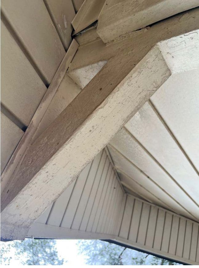
View of deteriorated LBP at Exterior Wall C – 45 degree supports
