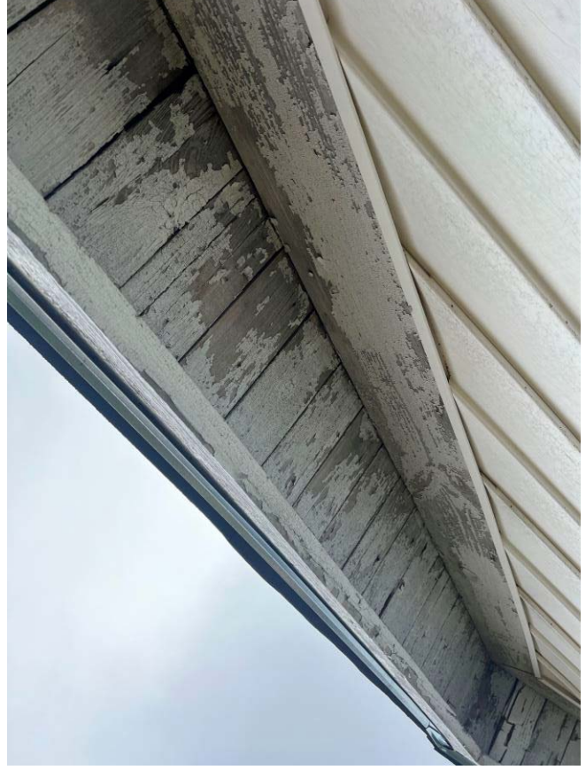
View of deteriorated LBP at Exterior Wall A - Fascia and Roof Deck
