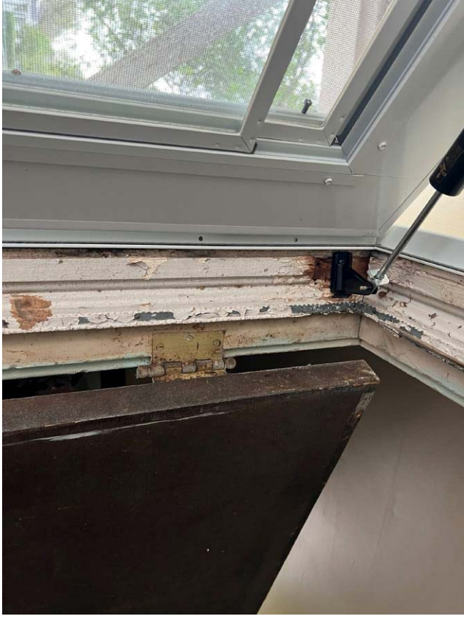
View of deteriorated LBP at Exterior Wall A – Door Frame.
