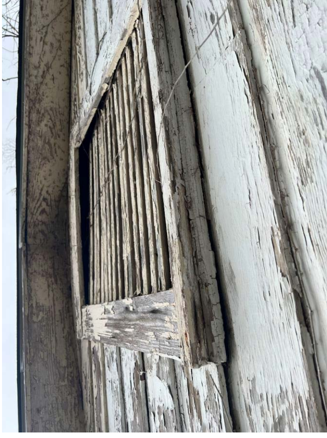
View of deteriorated LBP at Exterior Wall D – Gable Vent
