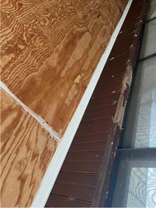
View of deteriorated LBP at Exterior Wall A – Porch Interior Wall
