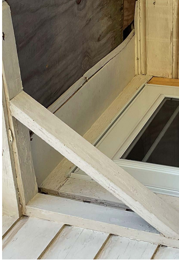
View of deteriorated LBP at Exterior Wall A - Porch Support
