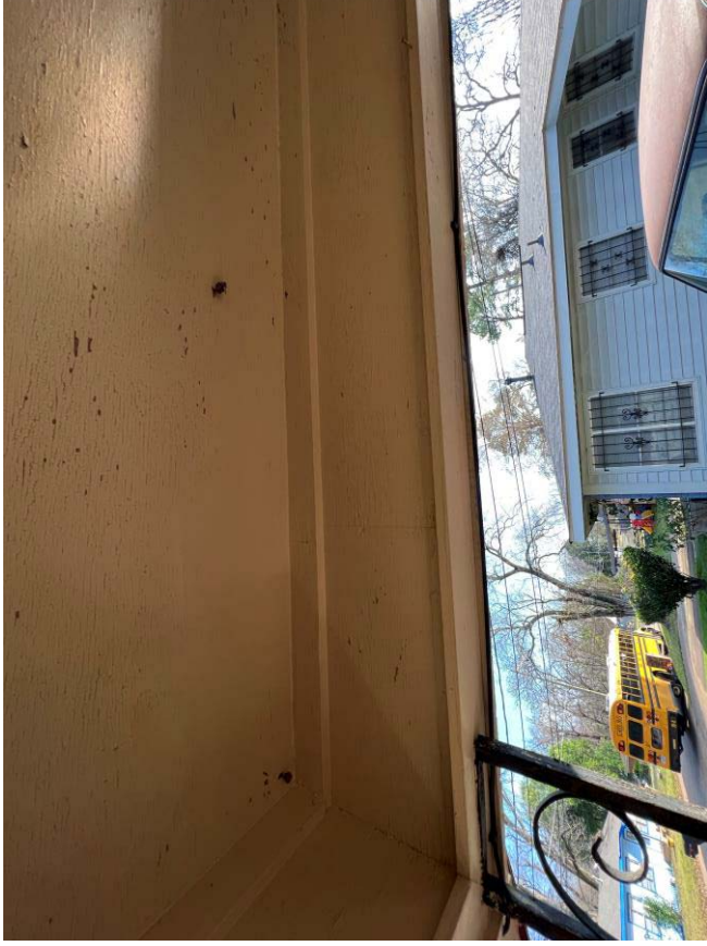
View of deteriorated LBP at Carport - Wall Cap.
