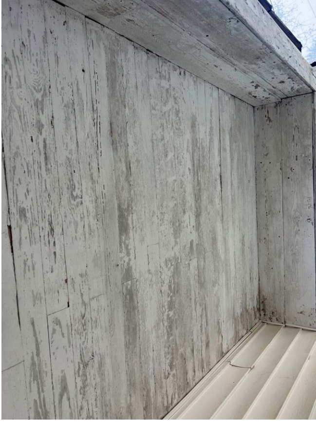
View of deteriorated LBP at Exterior Wall A - porch ceiling.
