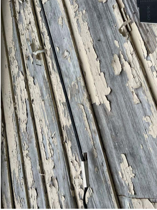
Representative view of deteriorated LBP at exterior walls.
