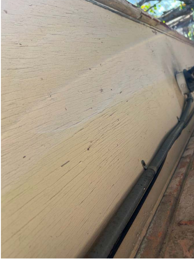
View of deteriorated LBP at Exterior Wall C - Soffit
