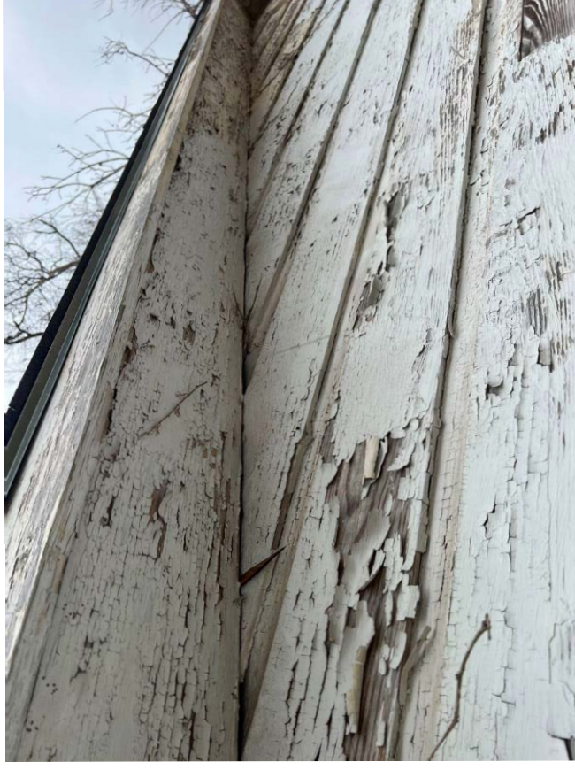
View of deteriorated LBP at Exterior Wall D - Roof Deck and Wall
