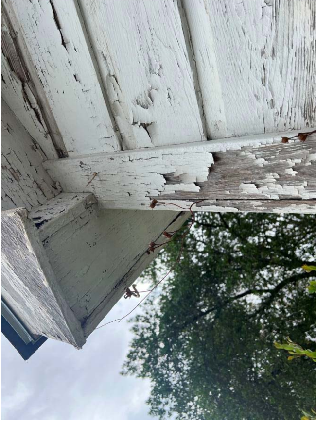
View of deteriorated LBP at Exterior Wall D - Trim
