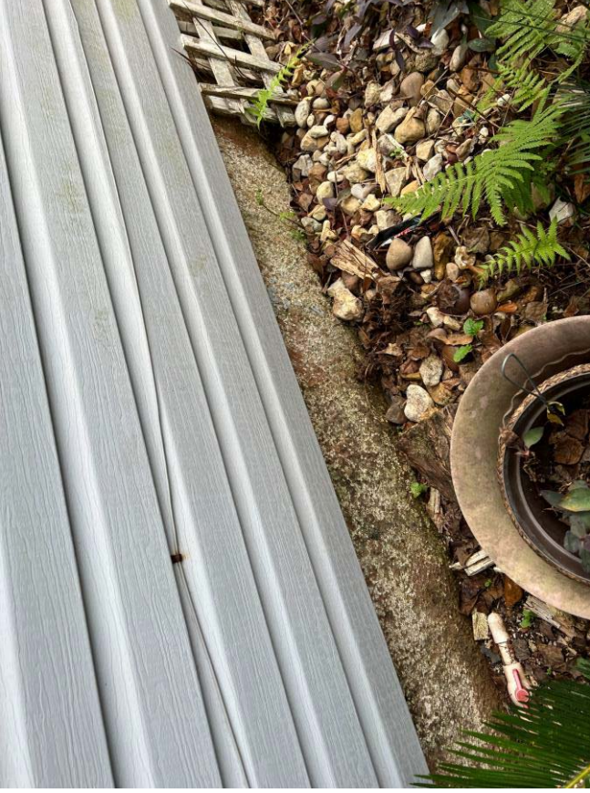
Representative view of deteriorated LBP on building skirt
