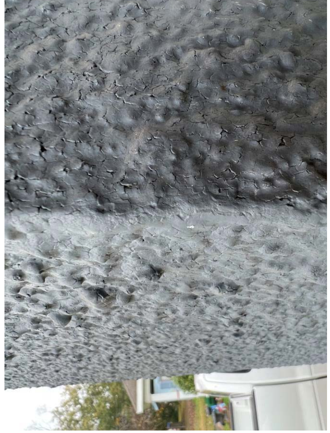
View of deteriorated LBP at Exterior Wall A - Porch Columns
