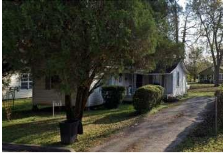
Front of House LAT 31°17'47.184"N LONG 92°25'39.2124" W
