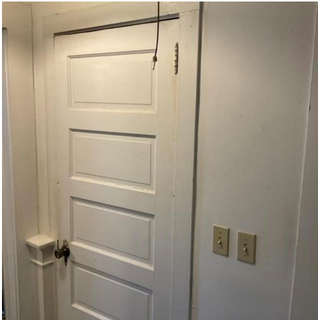
Hall - Friction and Impact surface with LBP
