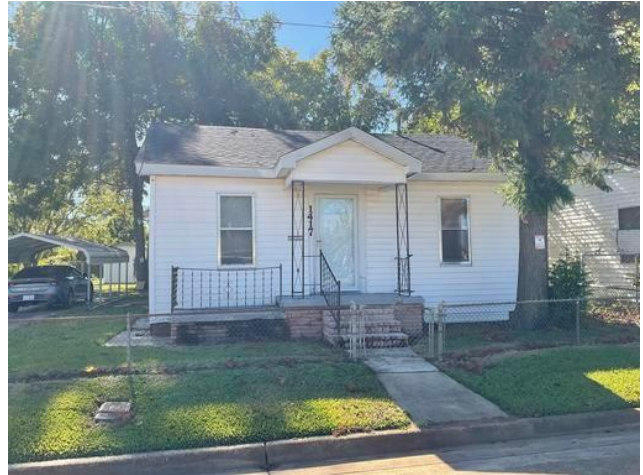
View of Exterior Wall A
