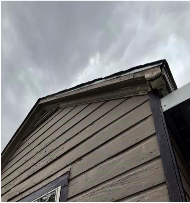
Exterior Wall A Fascia/Soffit: Deteriorated LBP
