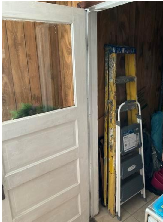
Kitchen Door Frame - Friction and impact surface with LBP
