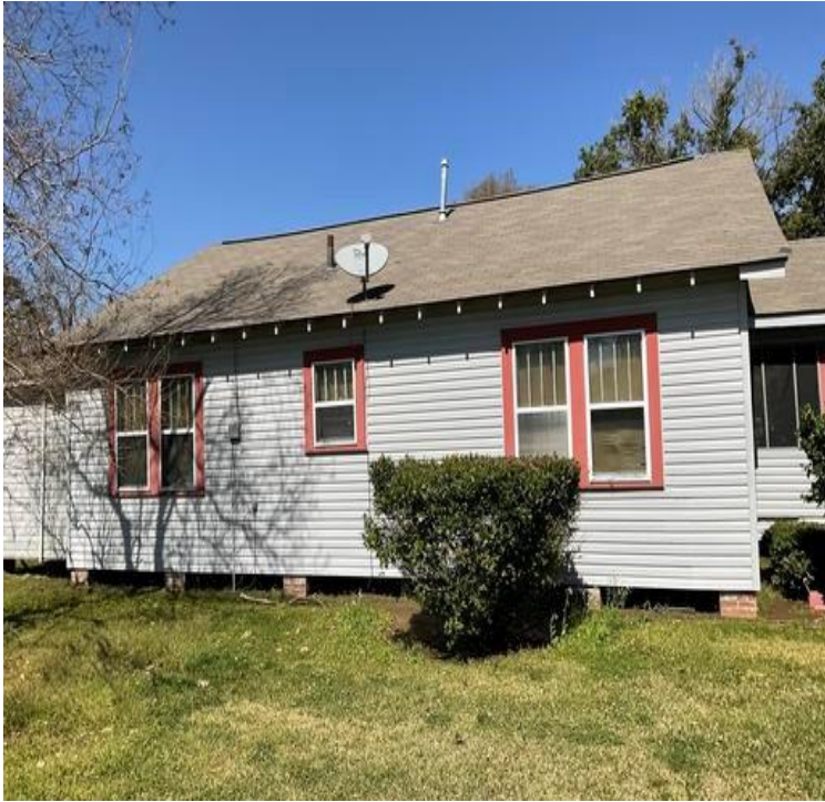
Exterior Wall B: View of covered windows
