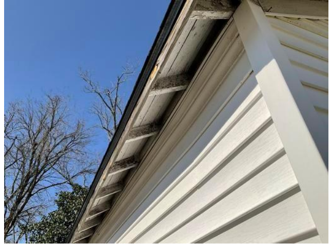
Exterior Wall B Roof Deck: Deteriorated LBP
