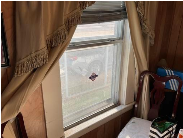
Dining Room Window - Friction and Impact Surface with LBP
