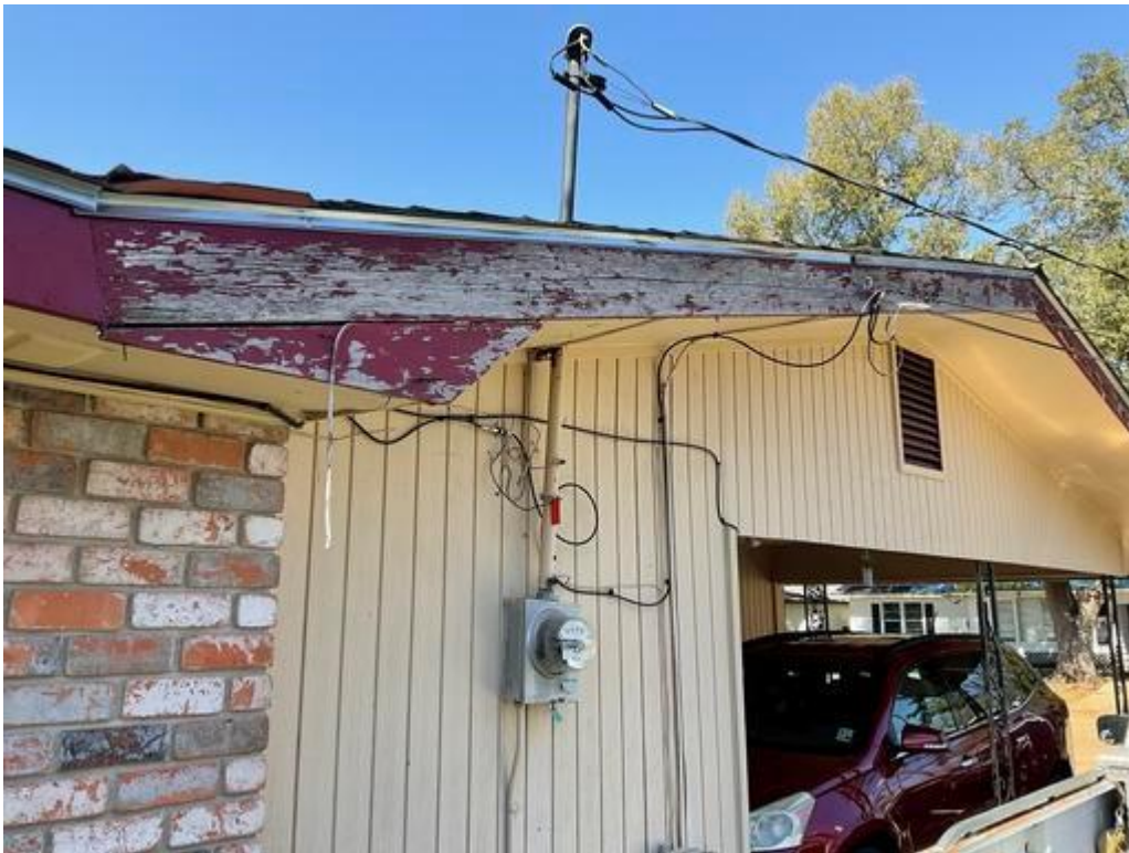
Exterior Wall B
