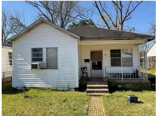
General View: Exterior Wall A
