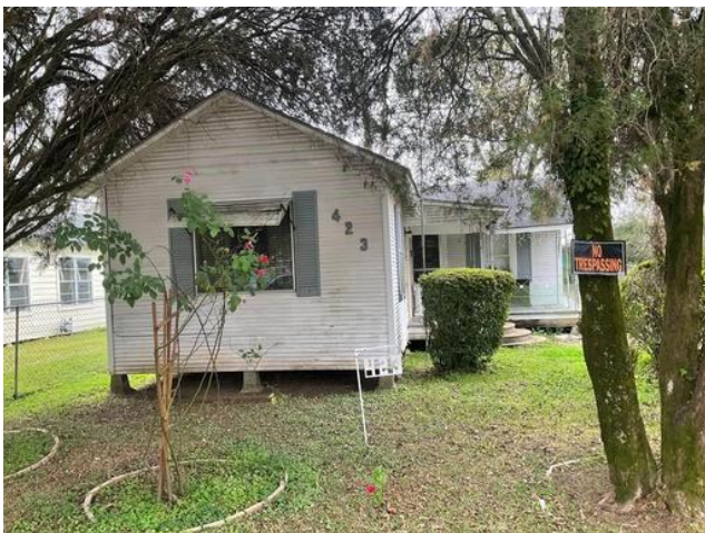
General View: Exterior Wall A
