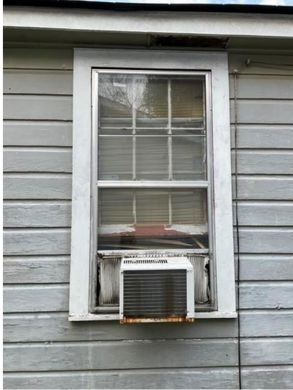
Exterior Wall B - Deteriorated LBP on casing
