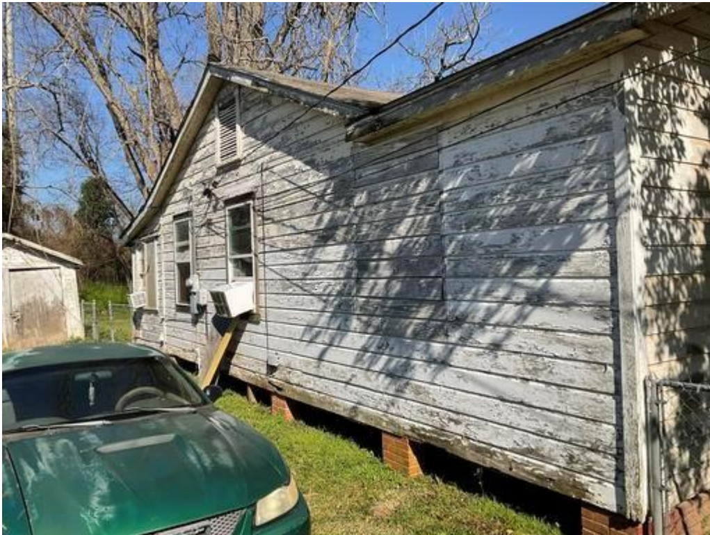
Exterior Wall B Wall: Deteriorated LBP
