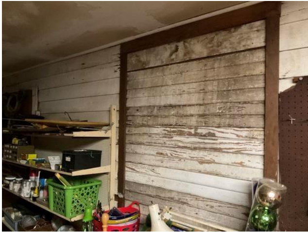
Utility Wall – Deteriorated LBP
