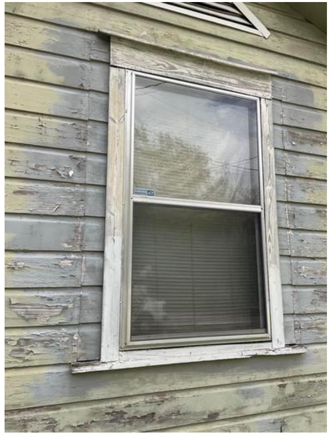
Exterior Wall A - Deteriorated LBP on casing
