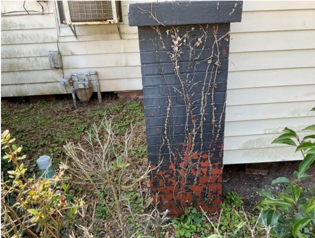
Exterior Wall A Brick Support Deteriorated LBP
