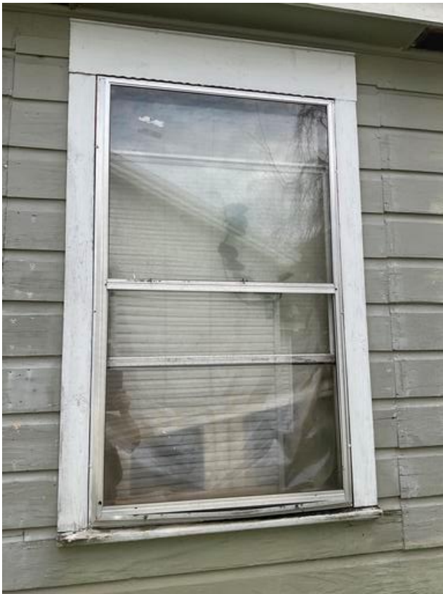
Exterior Wall D – Deteriorated LBP on casing
