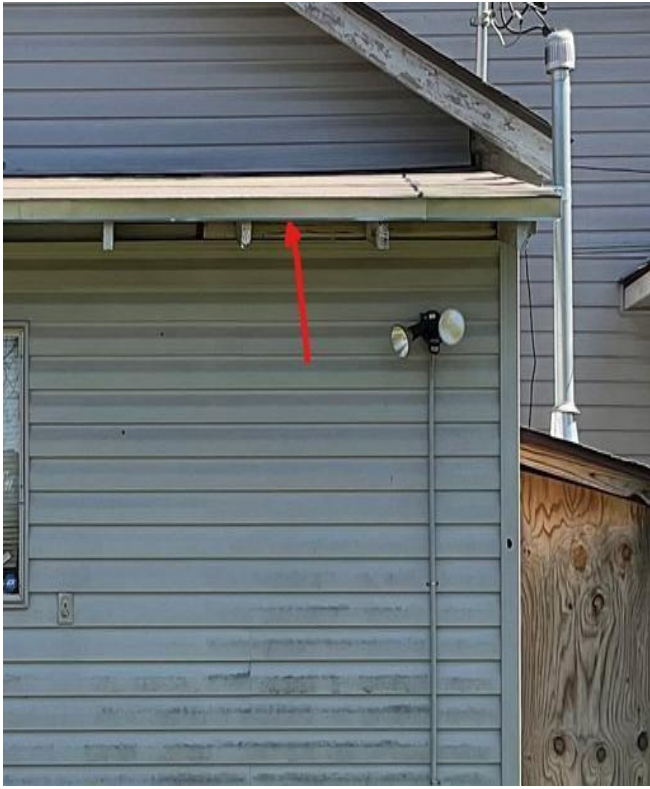
Exterior Wall C Wall: Deteriorated LBP
