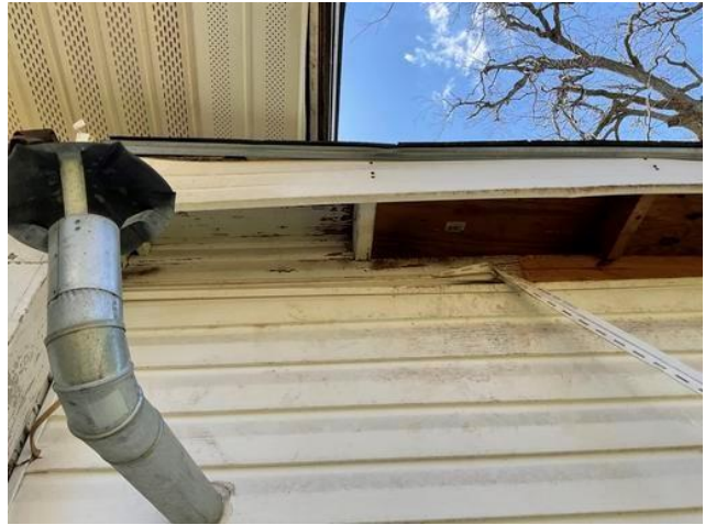
Exterior Wall D Roof Deck – Deteriorated LBP
