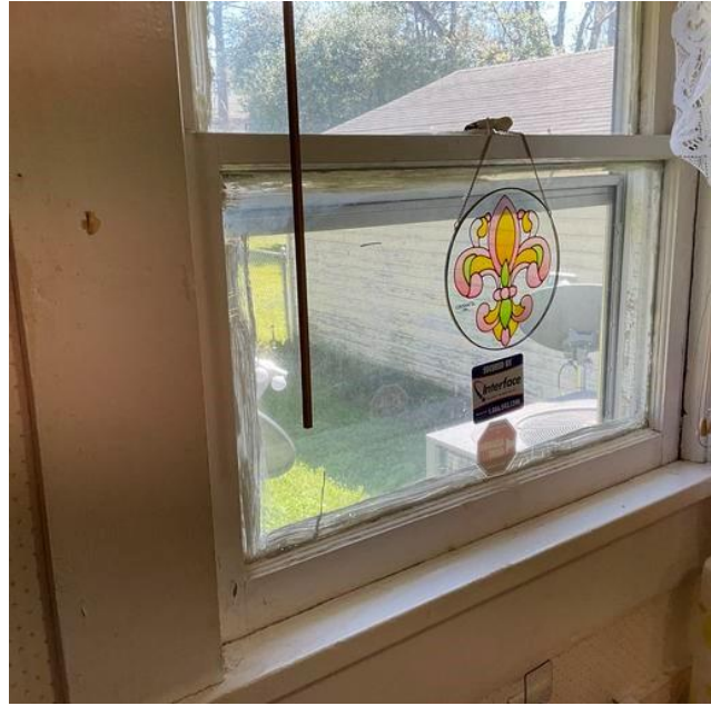
Bathroom 1 Window - Friction and Impact on surface with LBP
