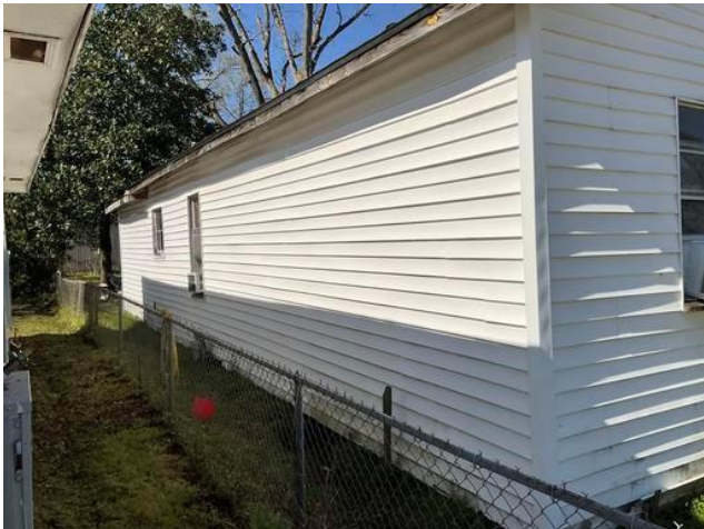
General View: Exterior Wall B
