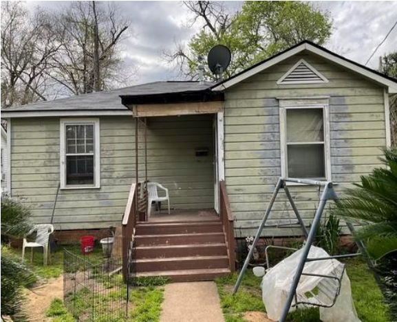
Exterior Wall A - Deteriorated LBP on Wall
