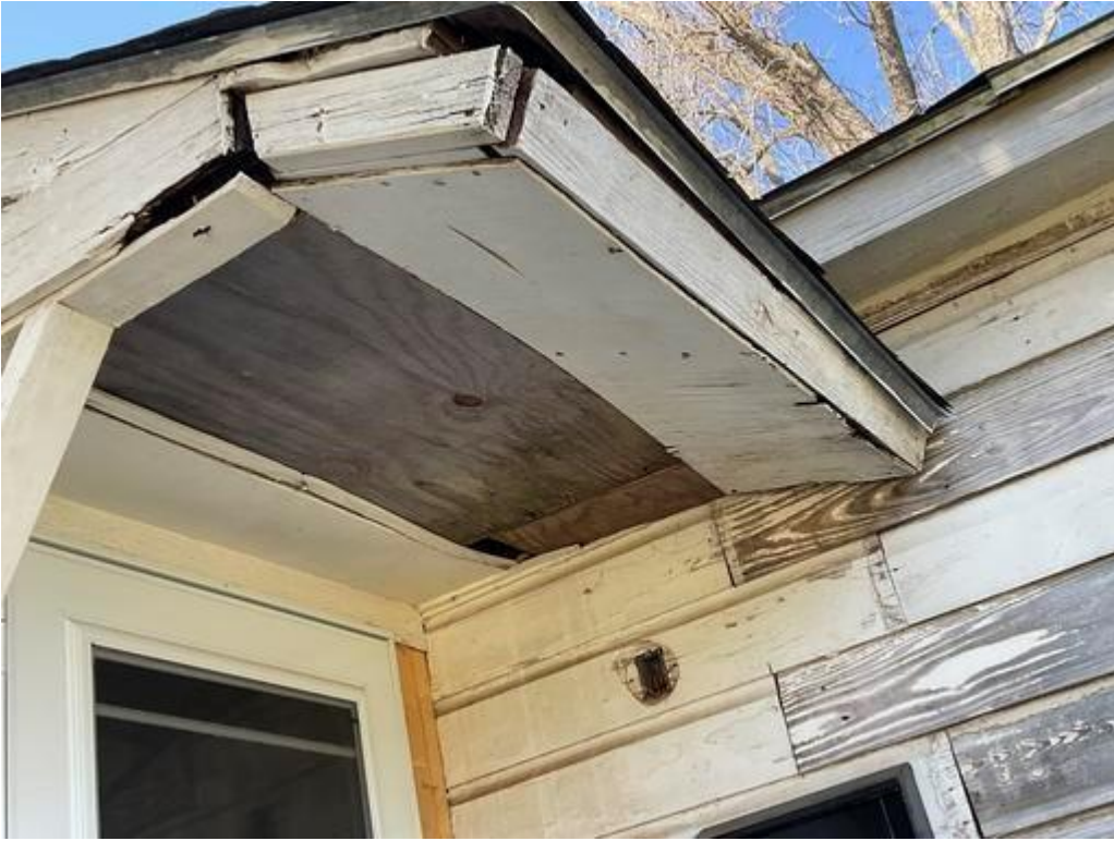
Exterior Wall A Porch: Deteriorated LBP
