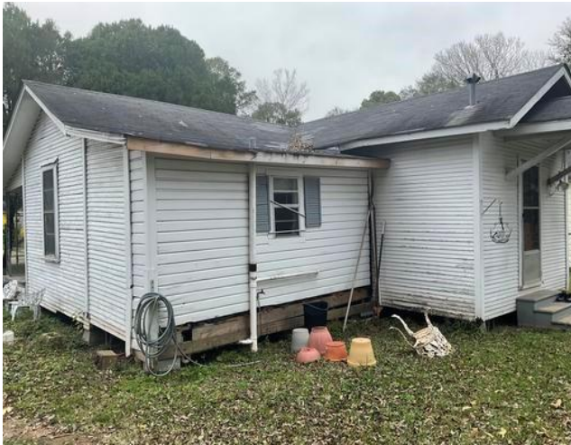
General View: Exterior Wall C
