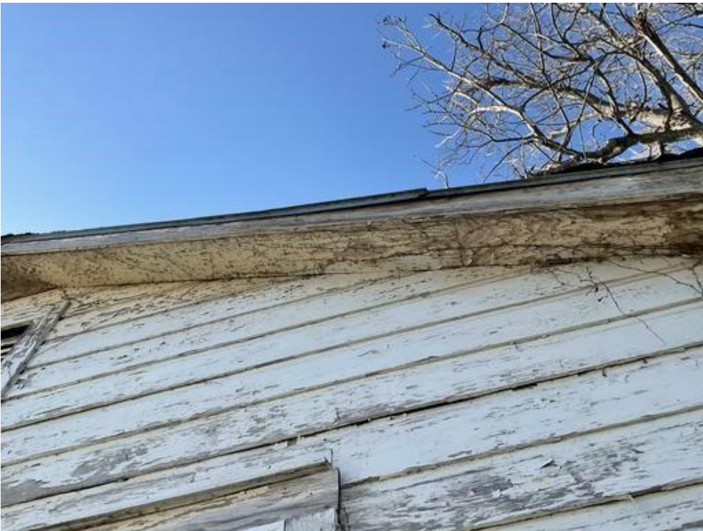
Exterior Wall D Roof Deck: Deteriorated LBP
