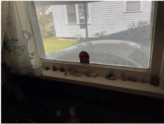
Kitchen Window - Friction and Impact on surface with LBP
