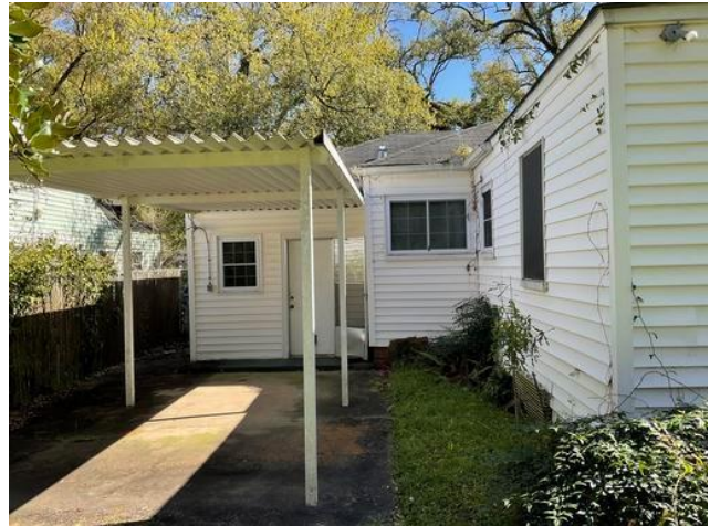
Additional View of Exterior Wall C
