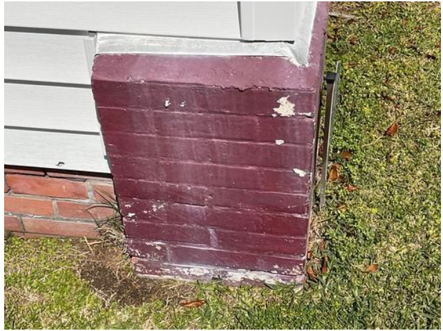
Exterior Wall A Brick Support – Deteriorated LBP
