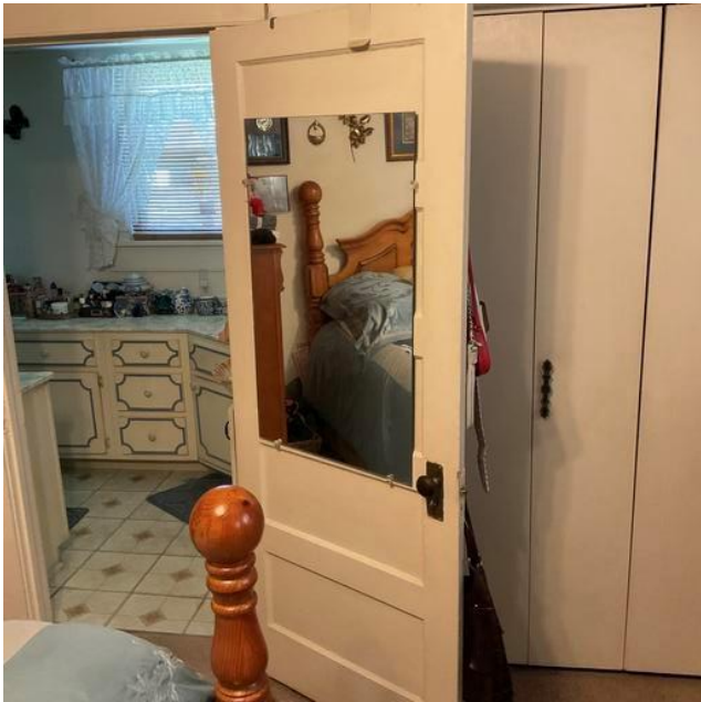
Bedroom 1 Door - Friction and Impact on surface with LBP
