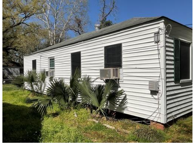
View of Exterior Wall B - Note covered windows.
