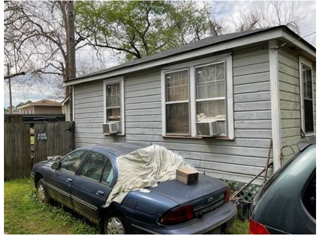
Exterior Wall B - General View
