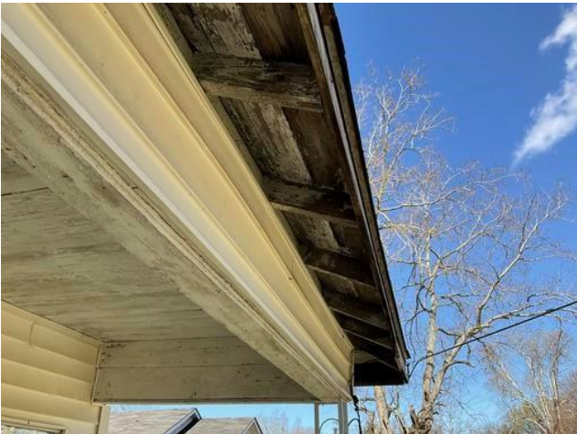
Exterior Wall A Rafters and Deck: Deteriorated LBP
