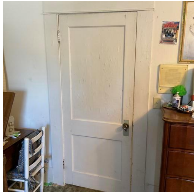
Bedroom 2 Door and Frame - Friction and Impact surface with LBP
