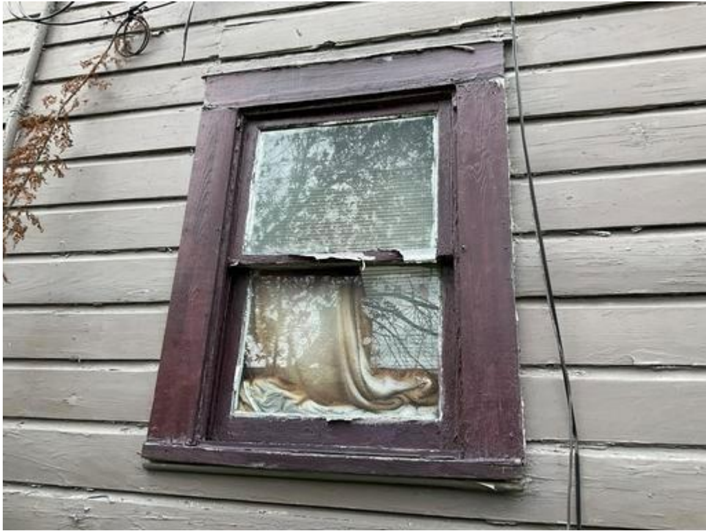
Exterior Wall B - Deteriorated LBP on window
