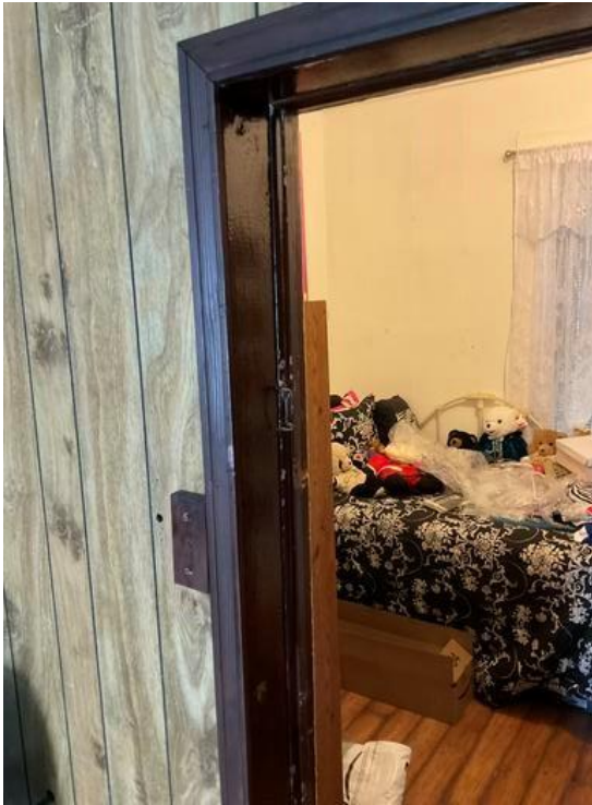
Bedroom 3 Door Frame - Friction and Impact surface with LBP
