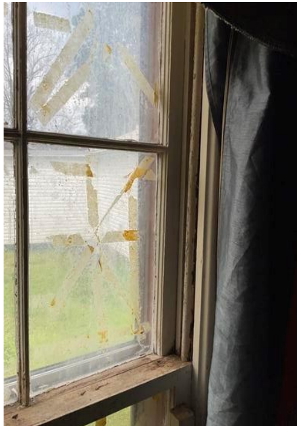
Kitchen - LBP on Window Frame
