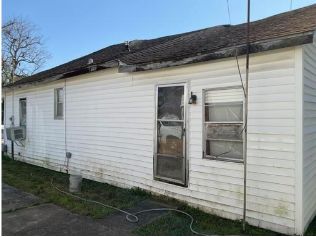
General View: Exterior Wall D
