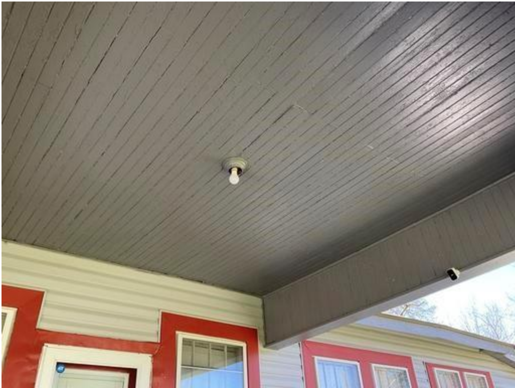
Exterior Wall D Canopy Roof: Deteriorated LBP
