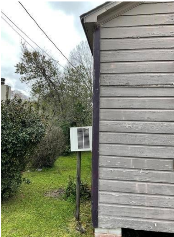
Exterior Wall A Trim: Deteriorated LBP
