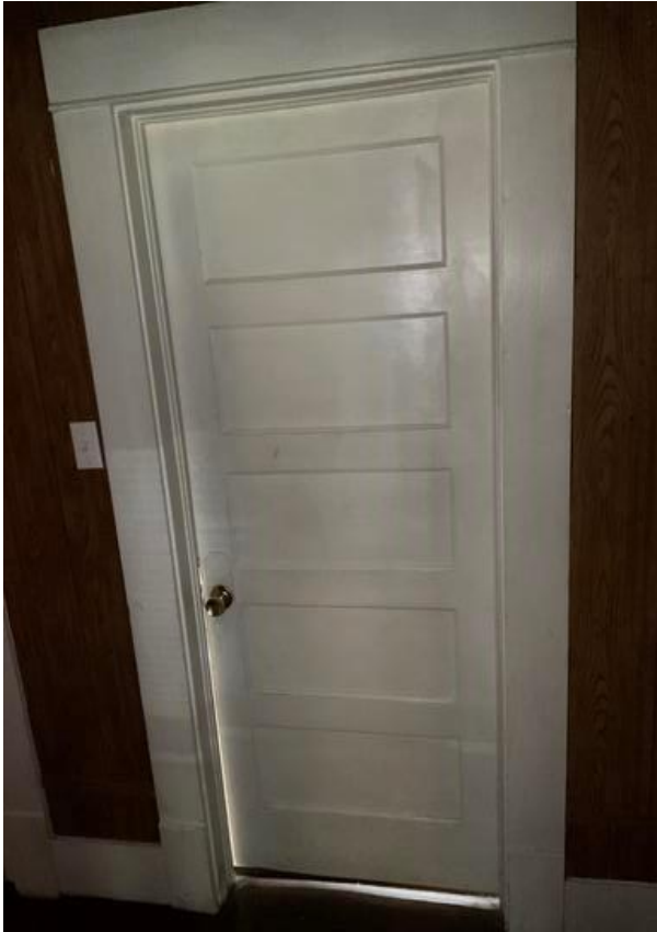
Bathroom/Hall Door: LBP Impact/Friction Surface
