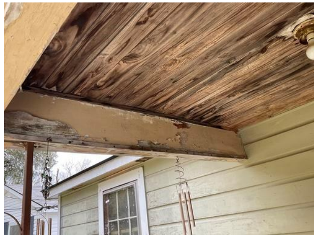
Exterior Wall A - Deteriorated LBP on wall cap
