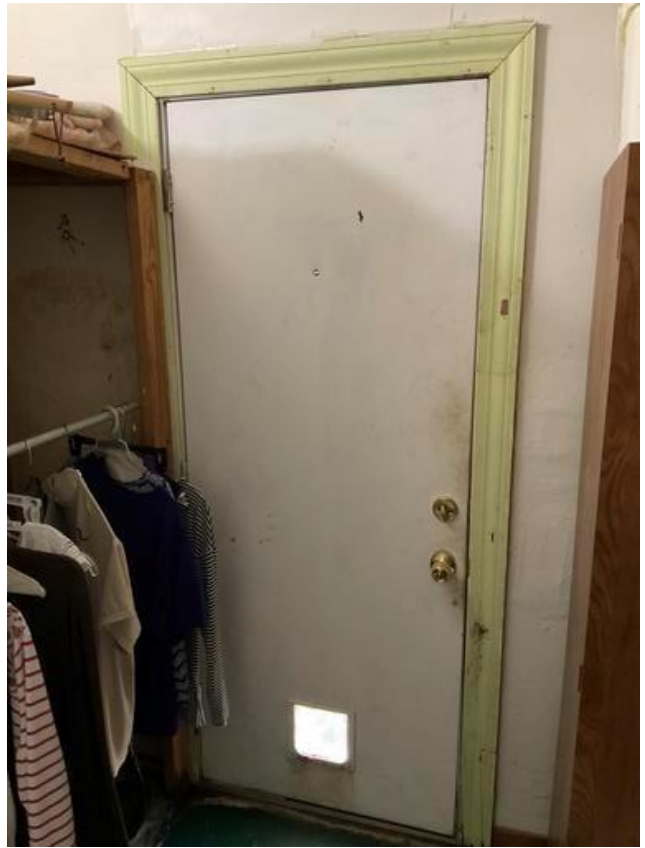
Utility Door and Casing - Friction and Impact Surface with LBP.
