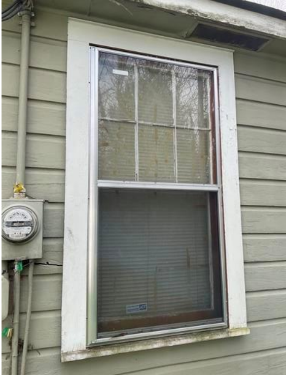
Exterior Wall D – Deteriorated LBP on soffit
