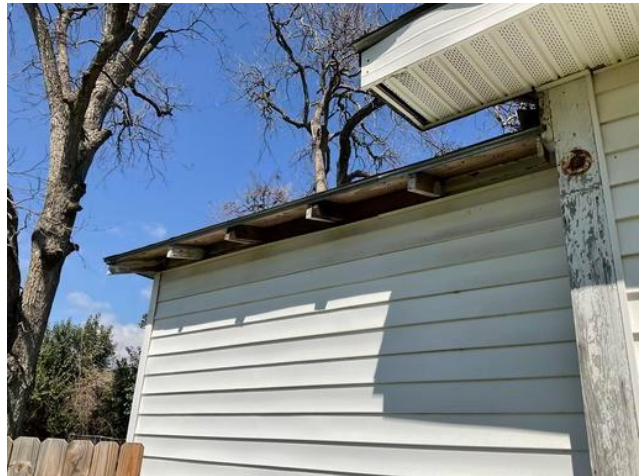
Exterior Wall B Trim – Deteriorated LBP
