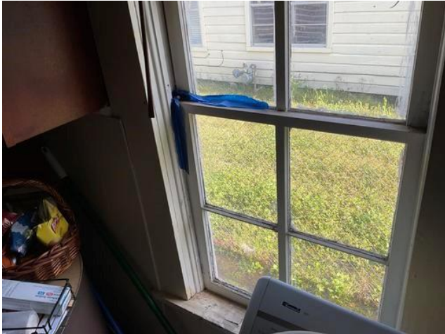
Kitchen Window: Friction/Impact Surface w/ LBP.
