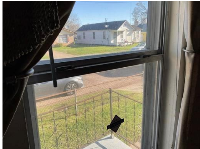
Living Room Window - Friction and Impact Surface with LBP
