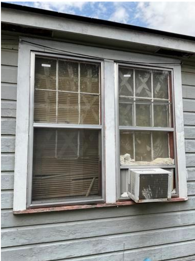
Exterior Wall B - Deteriorated LBP on casing
