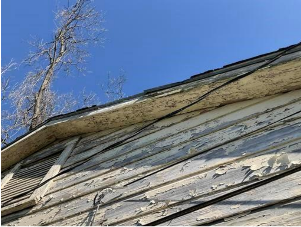
Exterior Wall B: Deteriorated LBP
