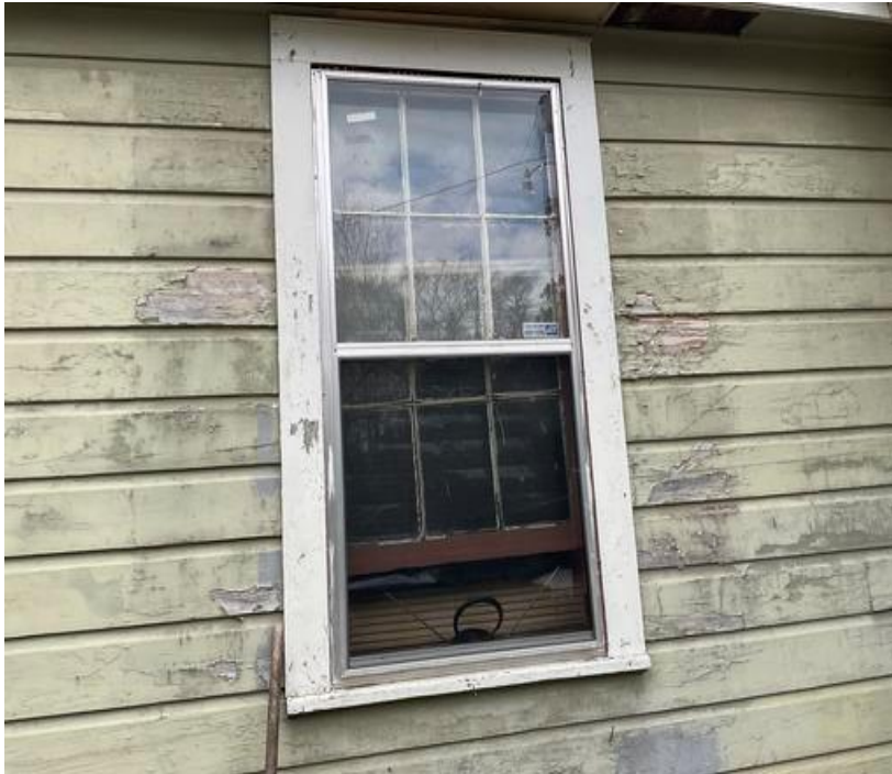
Exterior Wall A - Deteriorated LBP on casing
