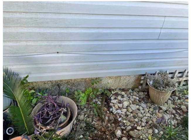
Exterior Wall B Skirt - Deteriorated LBP
