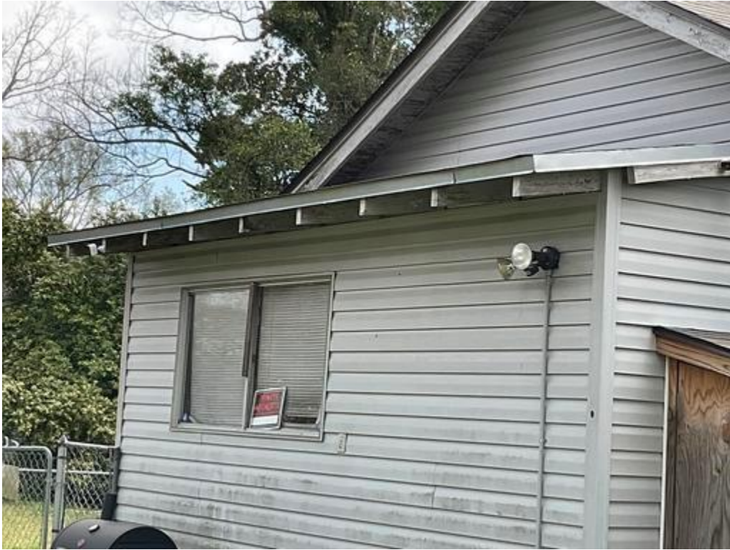
Exterior Wall C Rafter Tails: Deteriorated LBP
