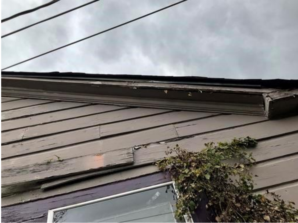
Exterior Wall B - Deteriorated LBP: Soffit
