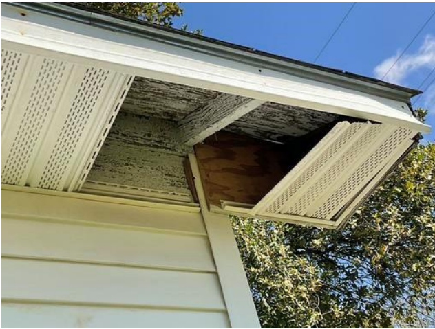
Exterior Wall B Rafter Tails – Deteriorated LBP
