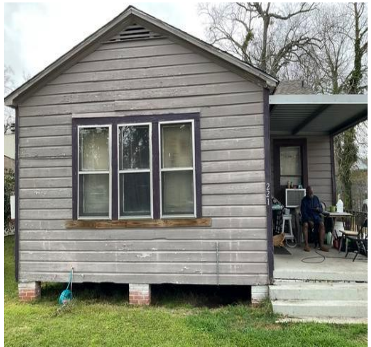
Exterior Wall A - Deteriorated LBP on wall.
