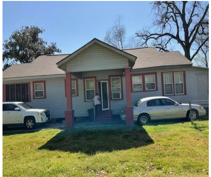
Exterior Wall D View of covered windows.
