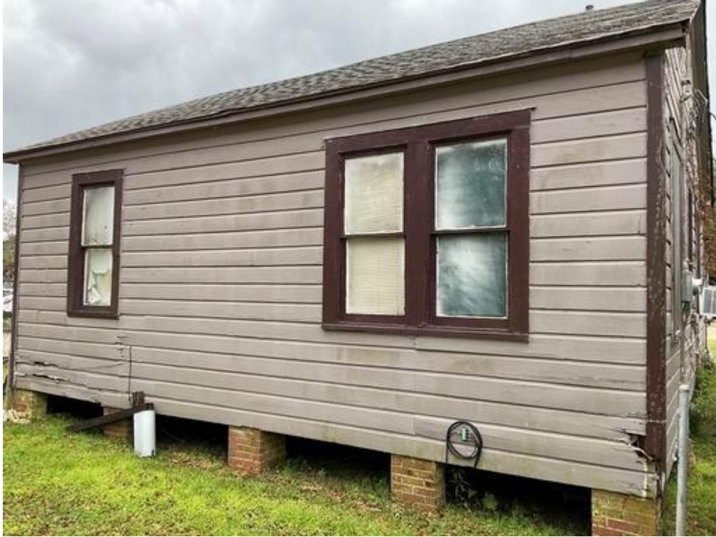
Exterior Wall C - Deteriorated LBP on windows/wall
