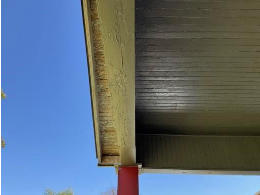
Exterior Wall D Wall Cap: Deteriorated LBP
