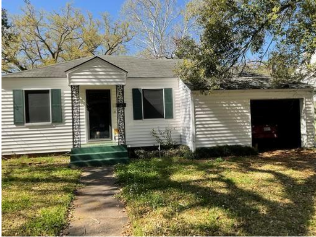
View of Exterior Wall A - Note covered windows.
