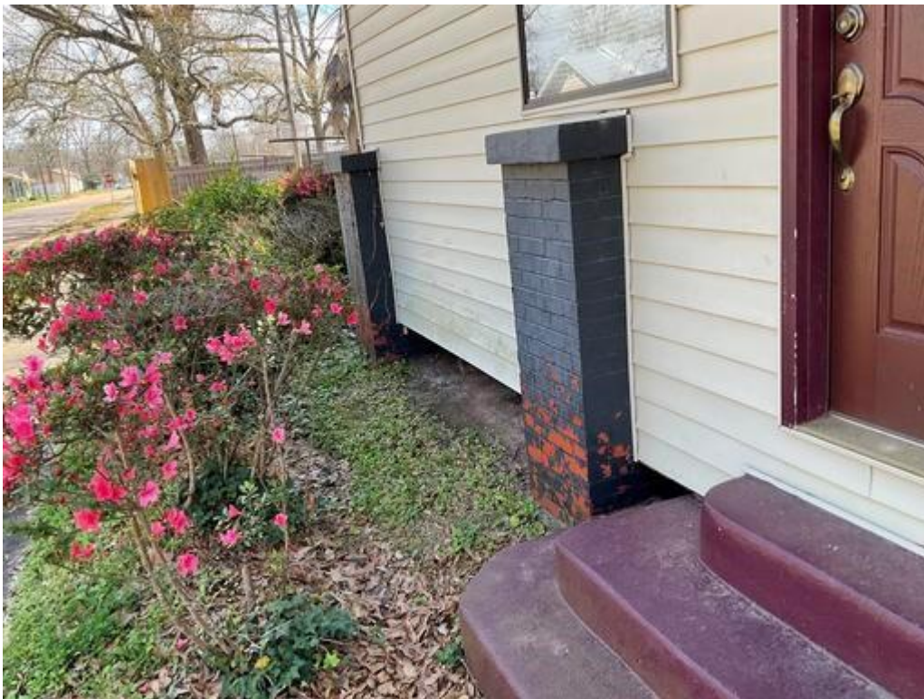
Exterior Wall B Brick Support Deteriorated LBP
