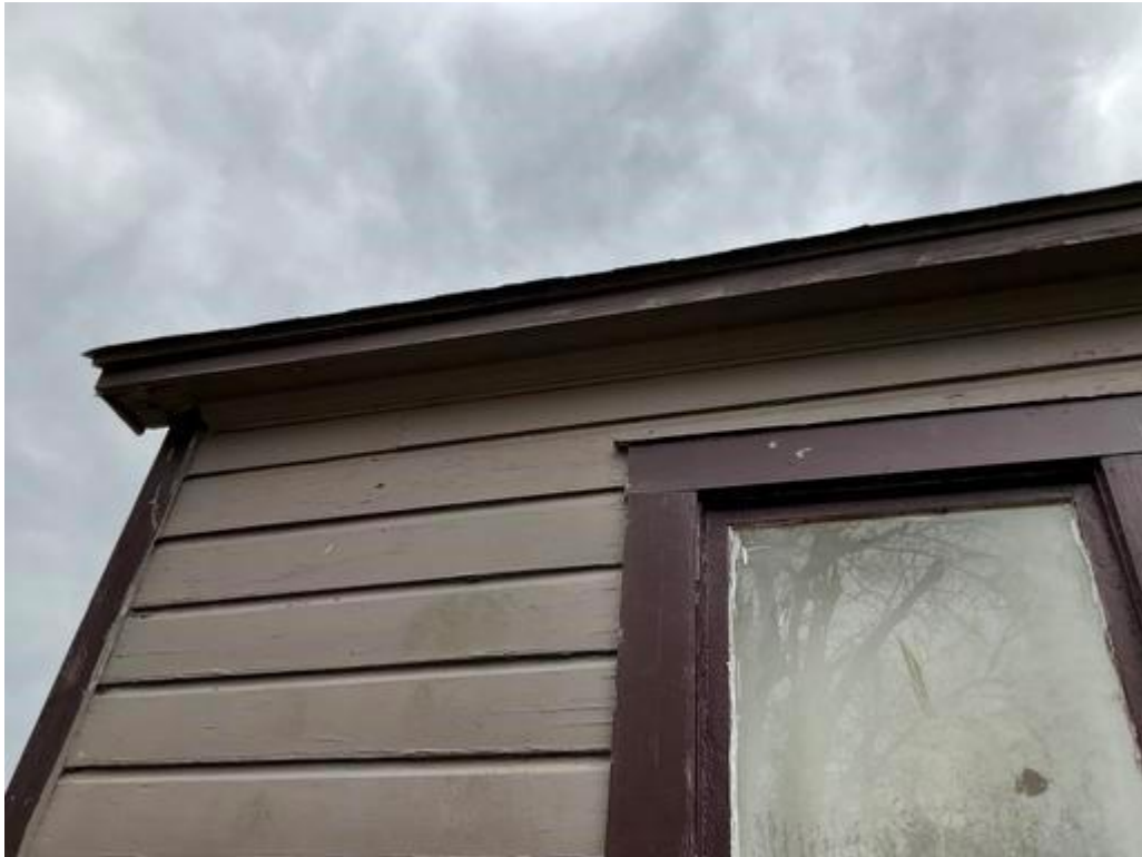
Exterior Wall C - Deteriorated LBP on soffit
