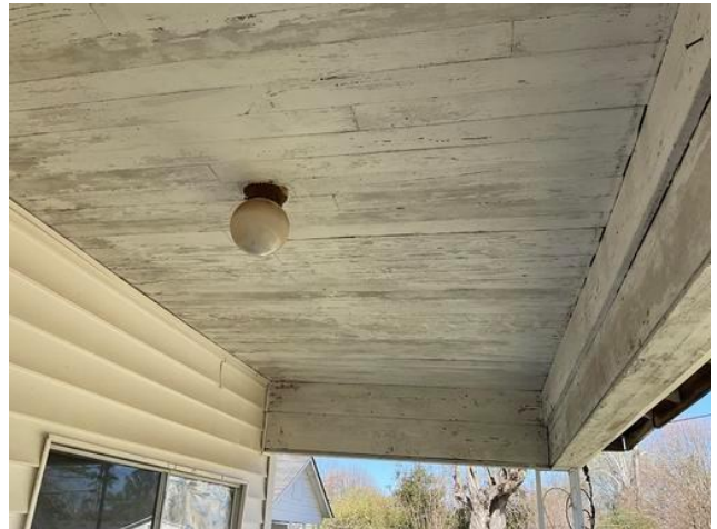
Exterior Wall A Porch Ceiling: Deteriorated LBP
