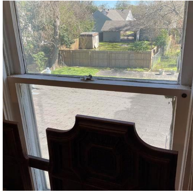
Bedroom 3 Window - Friction and Impact surface with LBP
