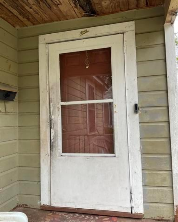
Exterior Wall A - Deteriorated LBP on casing
