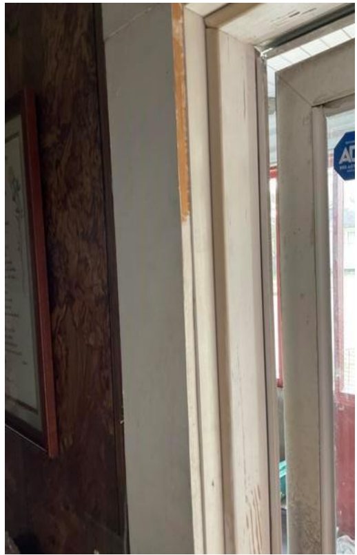
Living Room Door Casing: Deteriorated LBP
