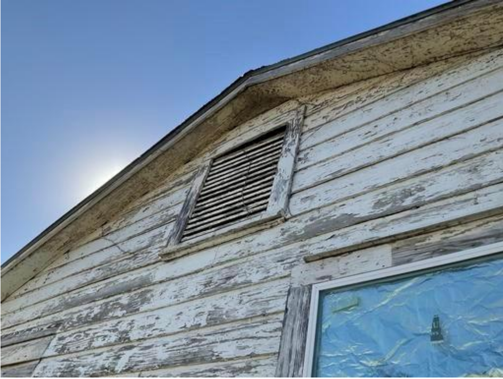
Exterior Wall D Gable Vent: Deteriorated LBP
