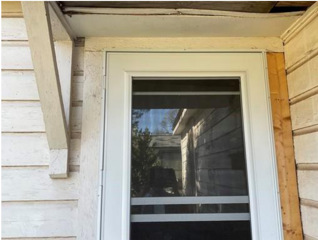
Exterior Wall A Door Frame: Deteriorated LBP
