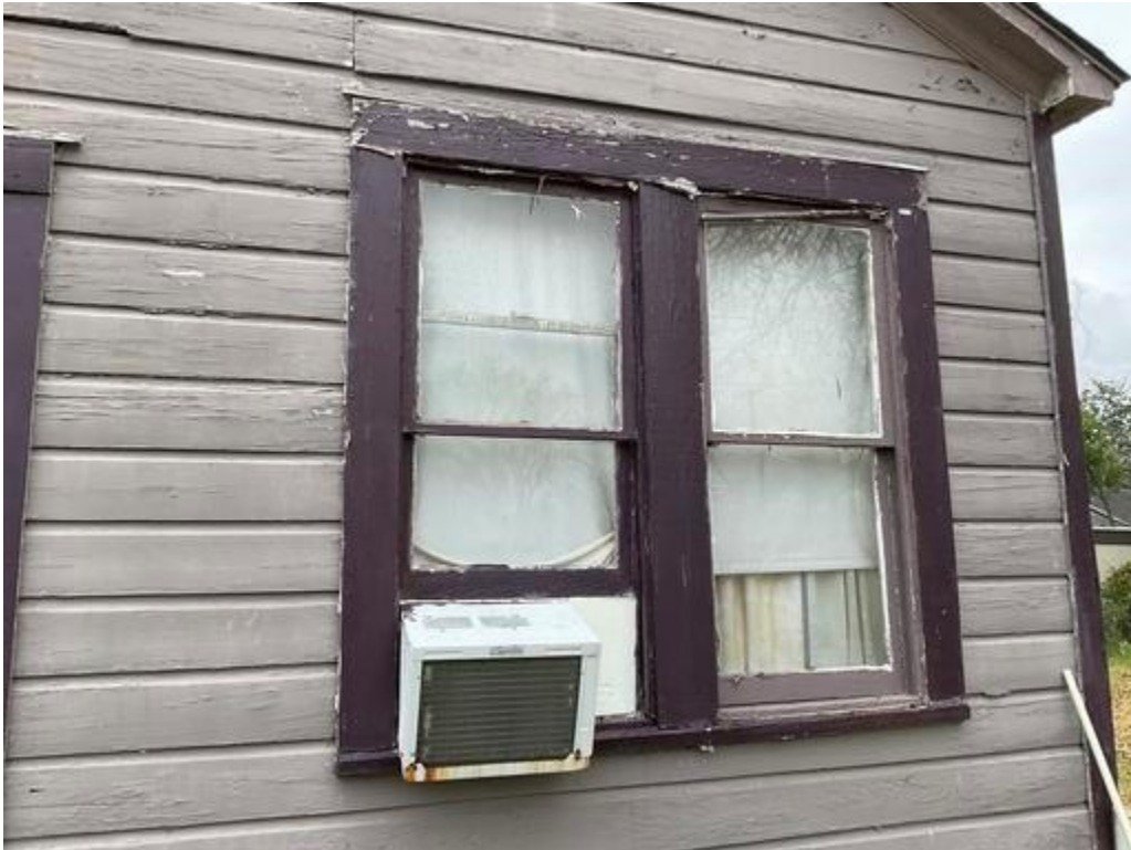
Exterior Wall D - Deteriorated LBP on windows/wall
