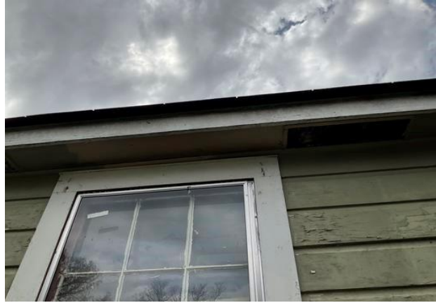
Exterior Wall B - Deteriorated LBP on soffit
