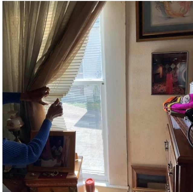
Bedroom 1 Window - Friction and Impact surface with LBP
