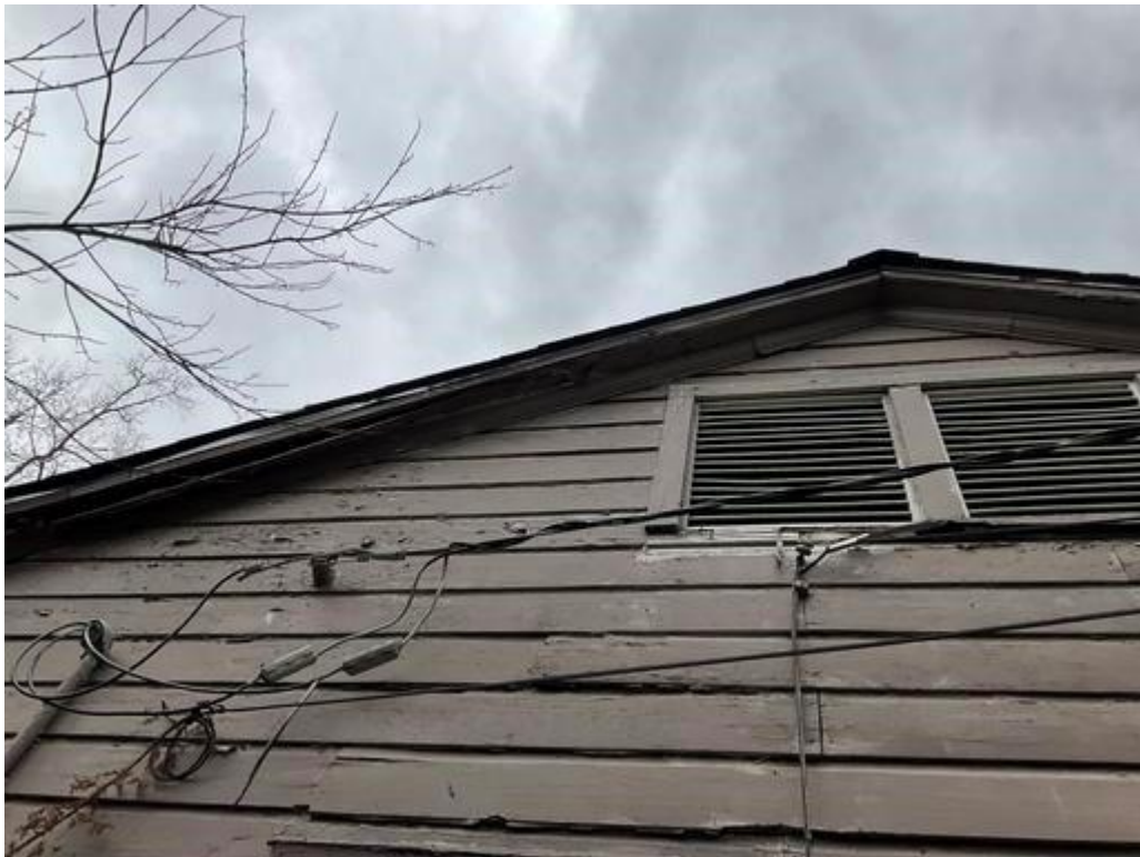
Exterior Wall B - Deteriorated LBP on gable vent
