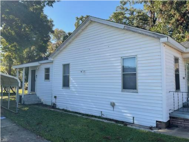
View of Exterior Wall B
