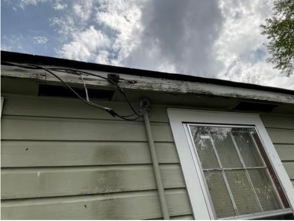
Exterior Wall D - Deteriorated LBP on fascia
