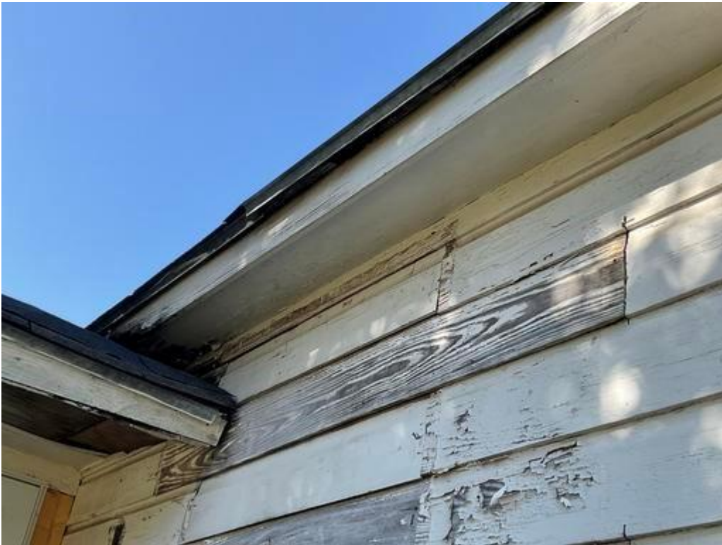
Exterior Wall A Roof Deck: Deteriorated LBP
