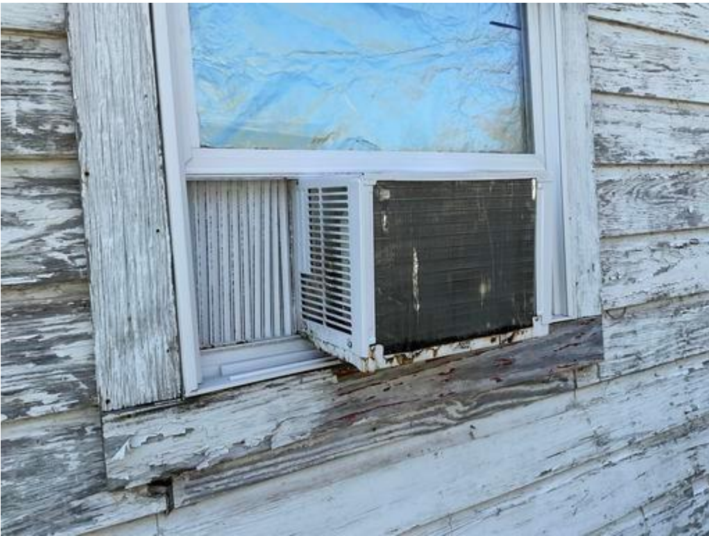
Exterior Wall D Window Casing: Deteriorated LBP
