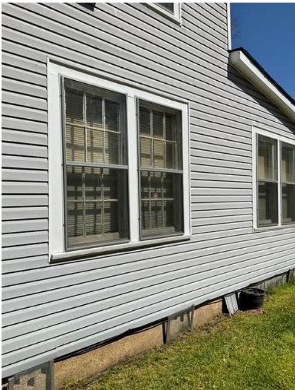
View of Exterior Wall D
