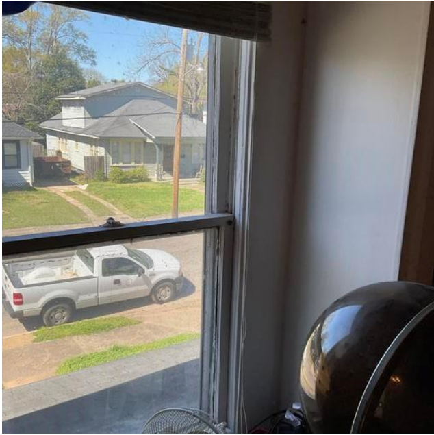
Bedroom 2 Window - Friction and Impact on surface with LBP
