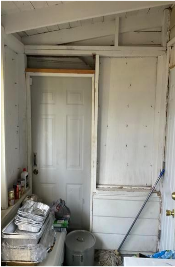
Utility Walls: Deteriorated LBP
