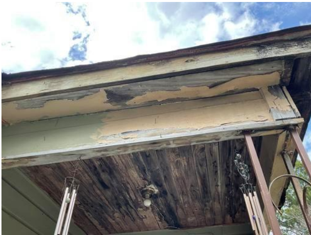
Exterior Wall A - Deteriorated LBP on soffit
