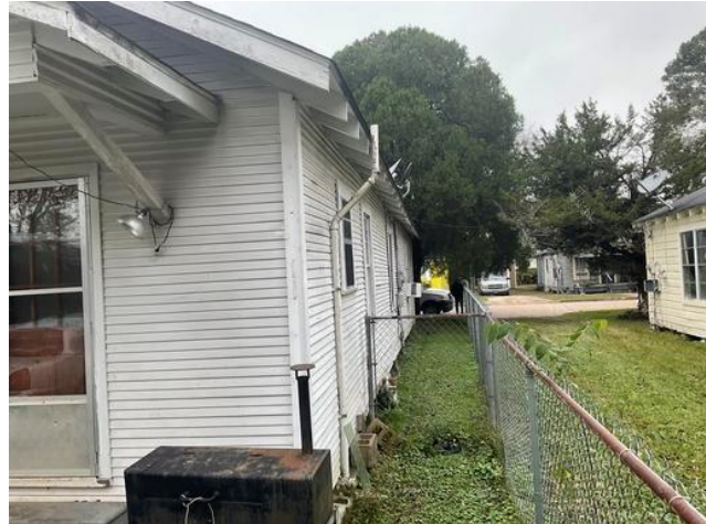
General View: Exterior Wall B
