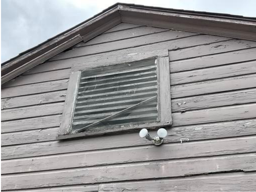
Exterior Wall D - Deteriorated LBP on gable vent
