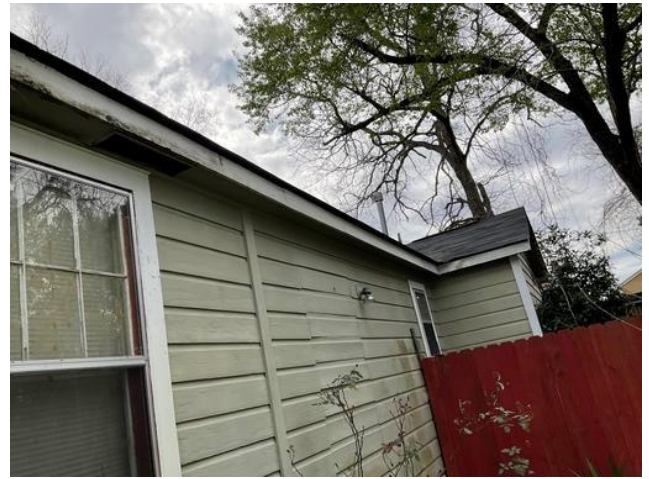
Exterior Wall D - General View
