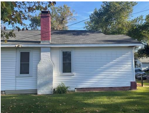
View of Exterior Wall B
