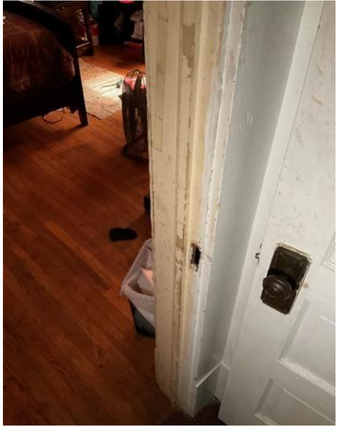
Bed 1 Door Frame: Deteriorated LBP
