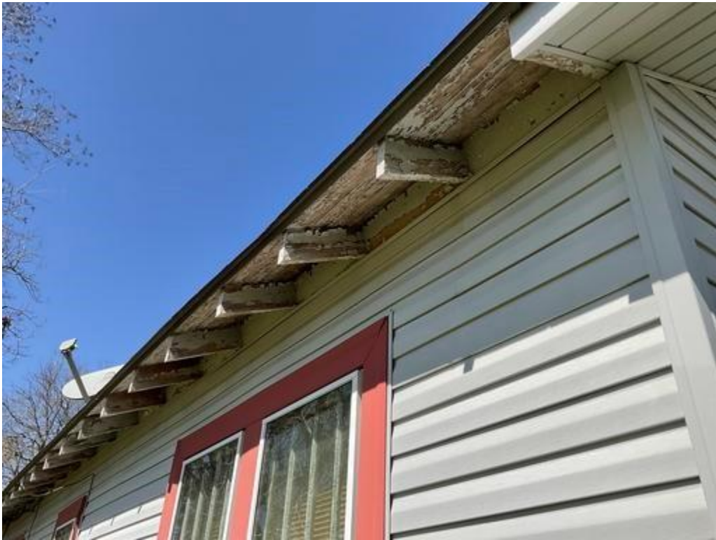
Exterior Wall B Rafter Tails: Deteriorated LBP
