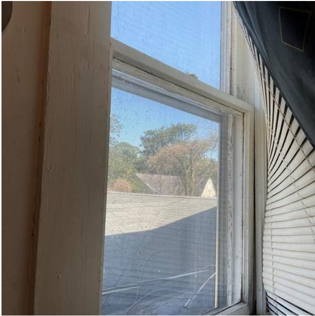
Stairwell Window - Friction and Impact surface with LBP
