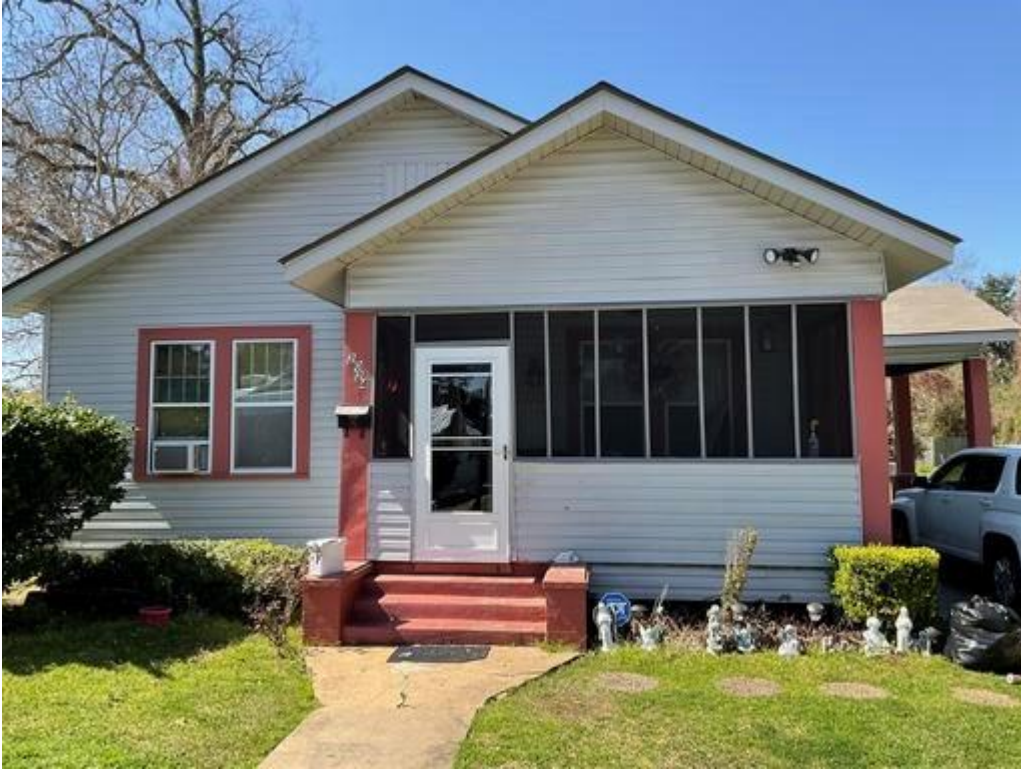
Exterior Wall A: View of covered windows.
