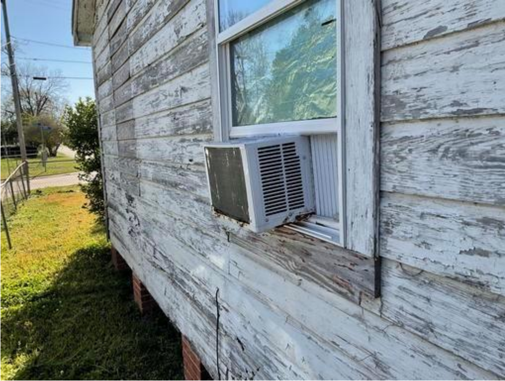
Exterior Wall D Window Casing: Deteriorated LBP
