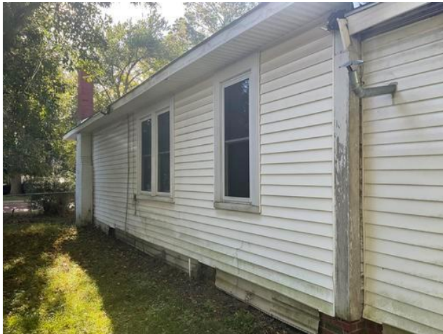
View of Exterior Wall D
