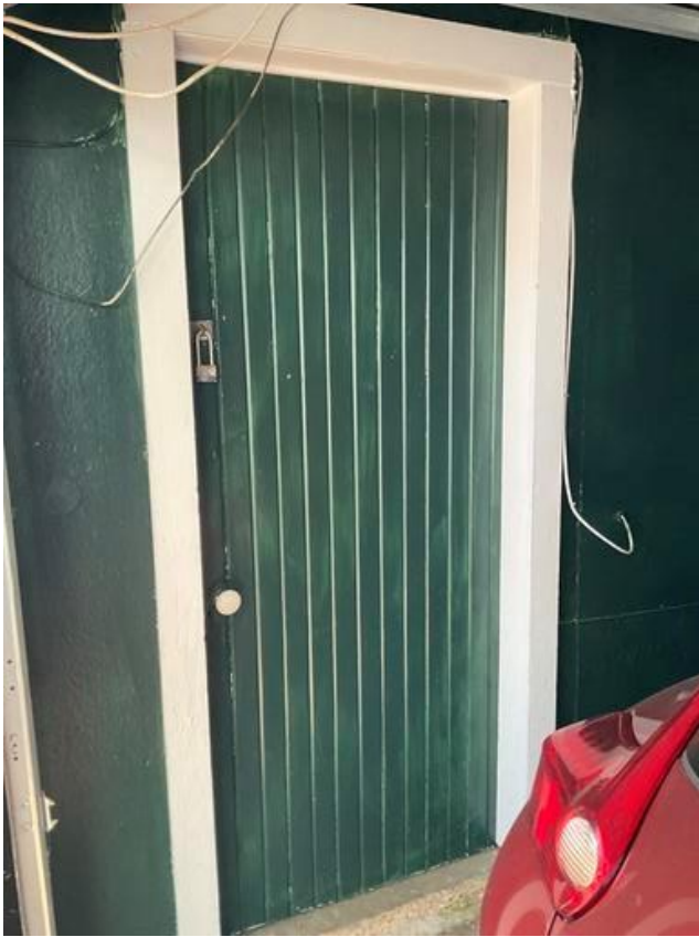
Garage Door and Casing - Friction and Impact Surface with LBP.
