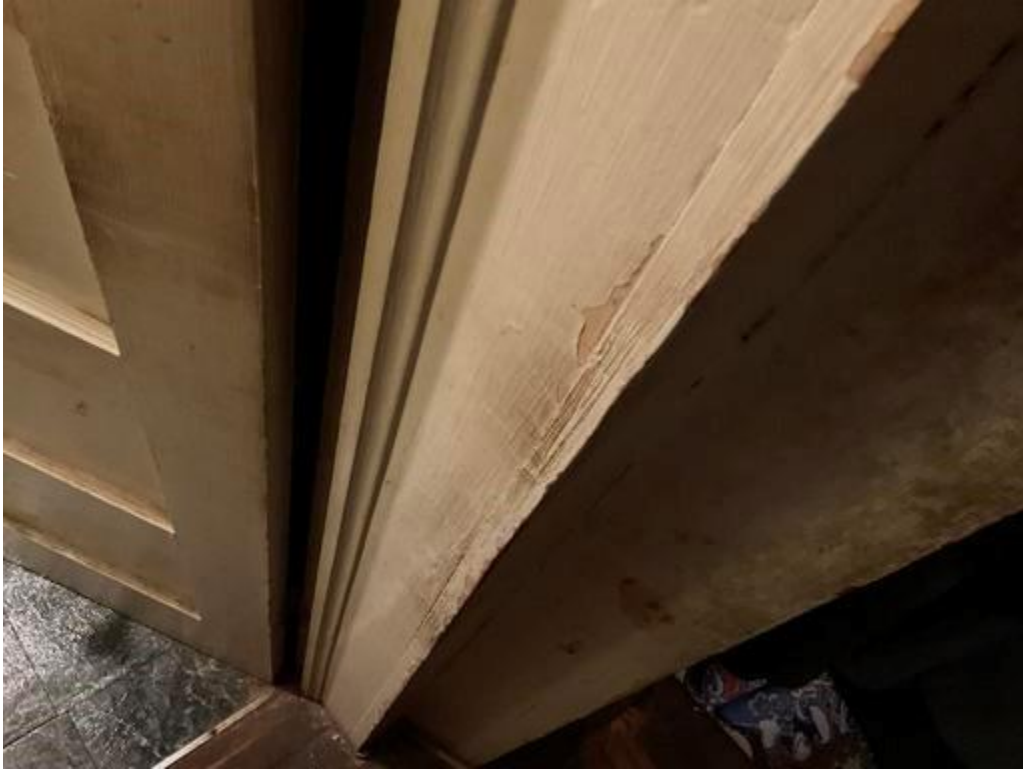
Bathroom 1 - Deteriorated LBP on casing
