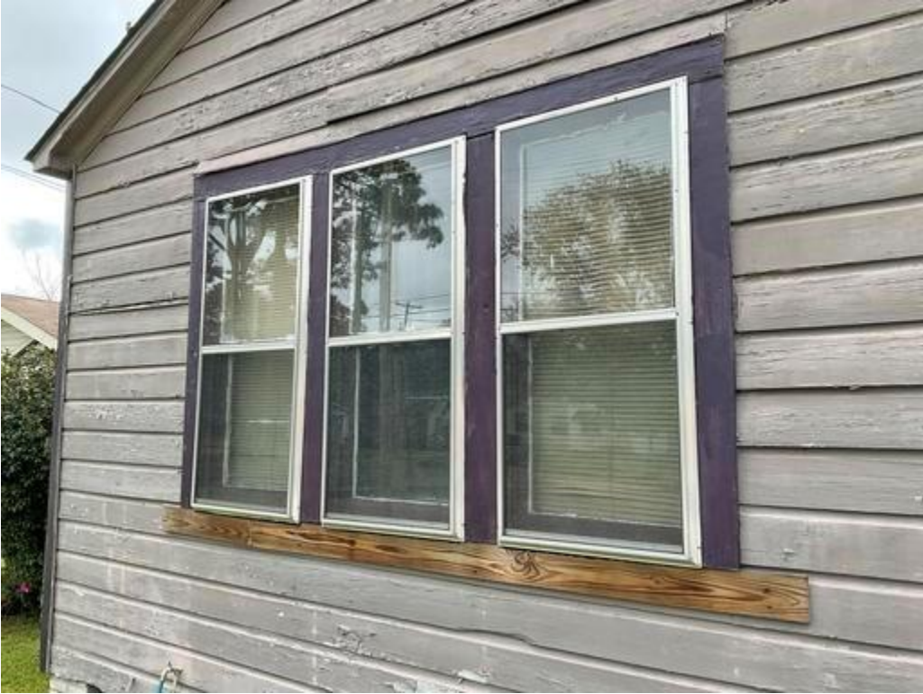
Exterior Wall C Windows - Deteriorated LBP
