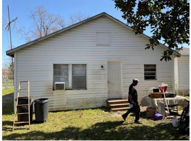
General View: Exterior Wall C
