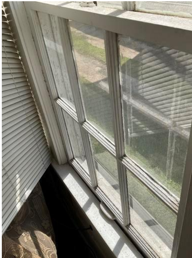
Living Room Window - Friction and Impact surface with LBP
