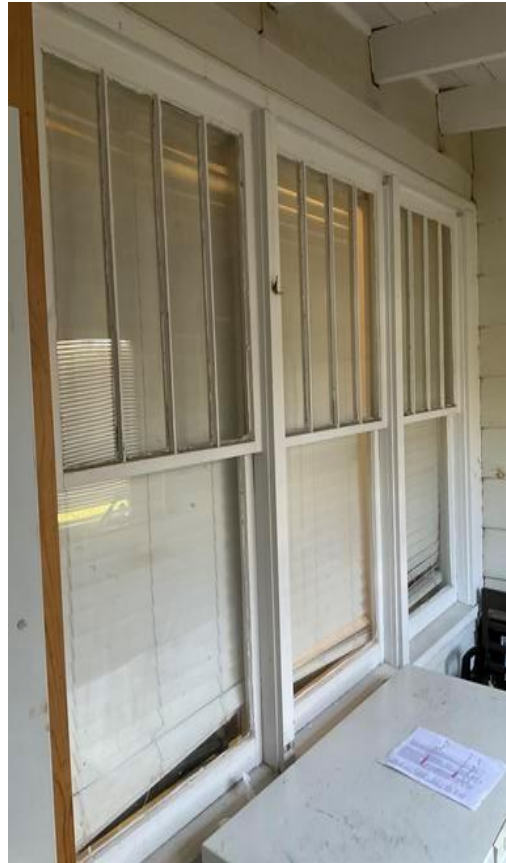
Utility Wood Windows: LBP Friction/Impact Surface
