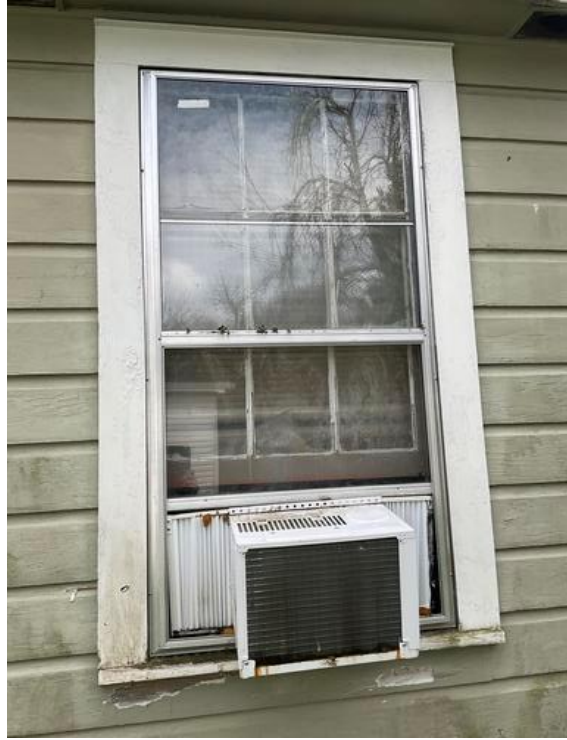
Exterior Wall D – Deteriorated LBP on casing
