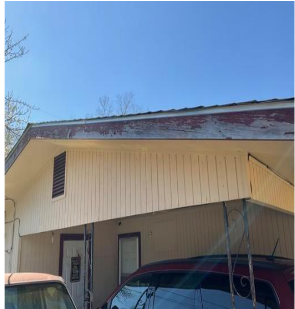
Exterior Wall D
