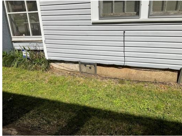
Exterior Wall D Skirt - Deteriorated LBP
