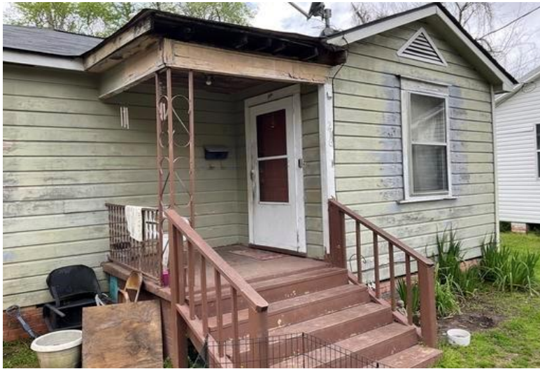
Exterior Wall A - General view of porch.
