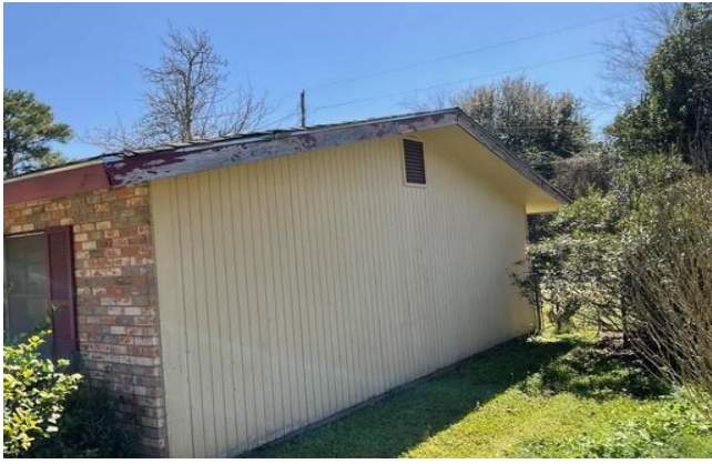
Deteriorated paint on wall
