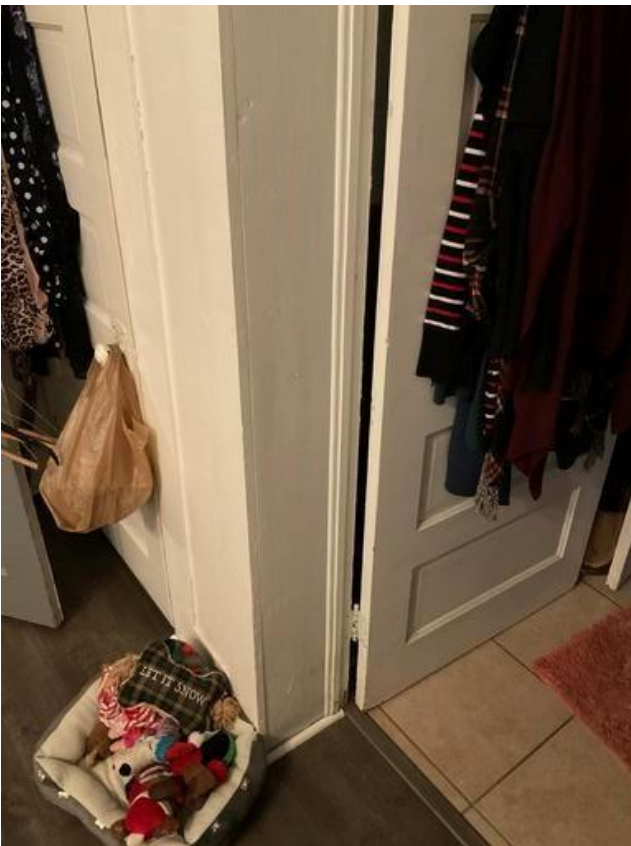
Bedroom 1 Door and Frame - Friction and Impact surface with LBP.
