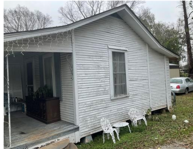
General View: Exterior Wall D
