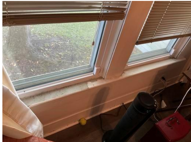
Bedroom 1 Windows - Friction and Impact Surfaces
