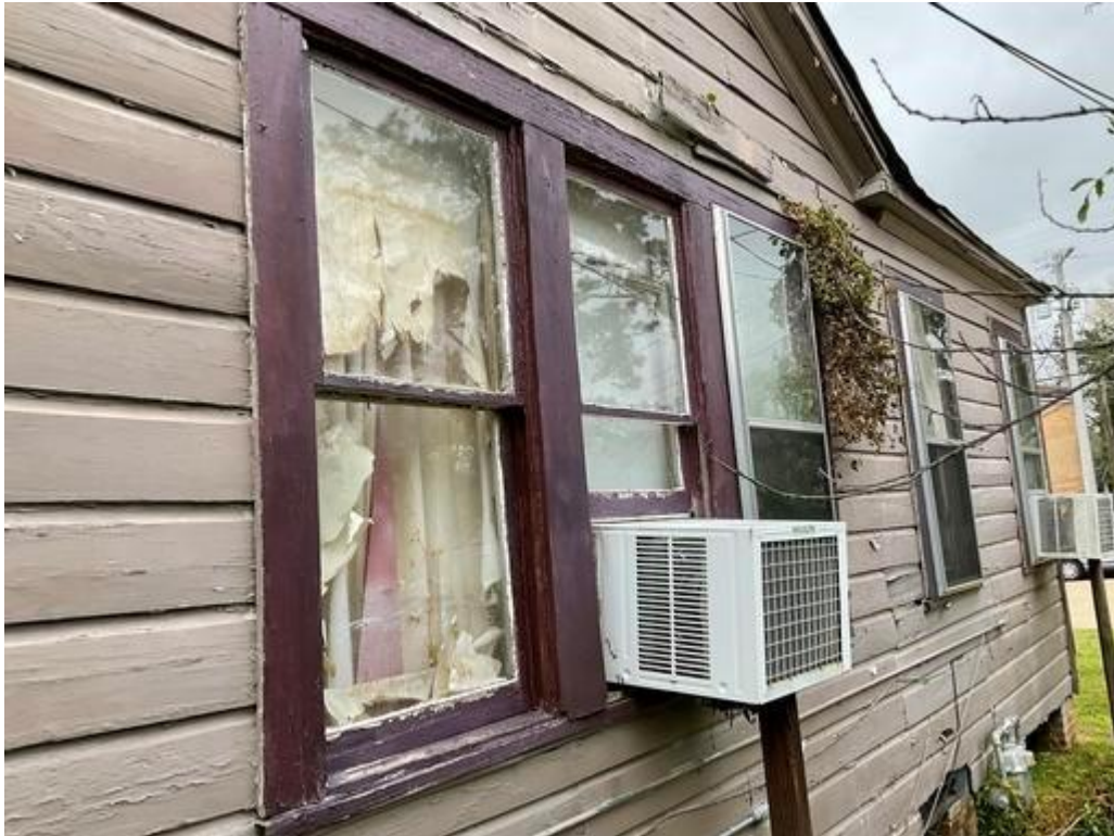
Exterior Wall B - Deteriorated LBP on windows/wall
