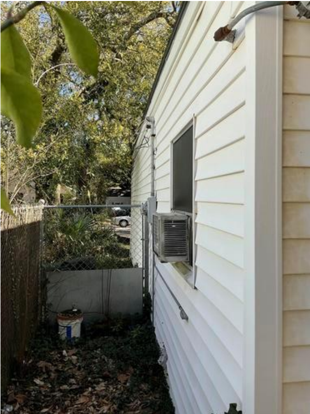
View of Exterior Wall D.
