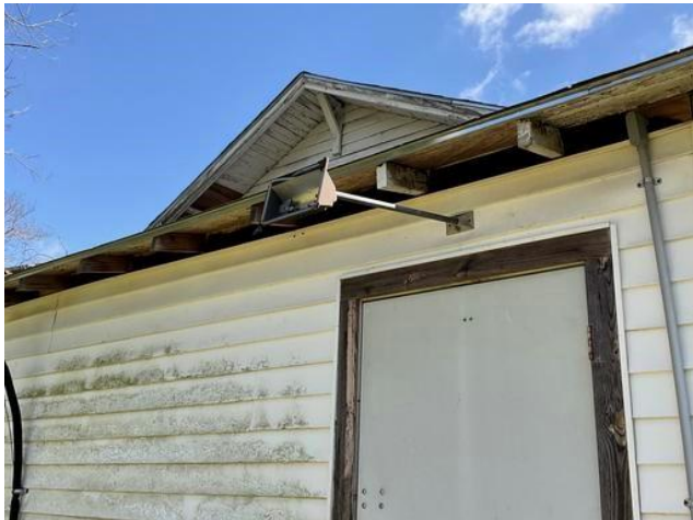
Exterior Wall C Rafter Tails – Deteriorated LBP
