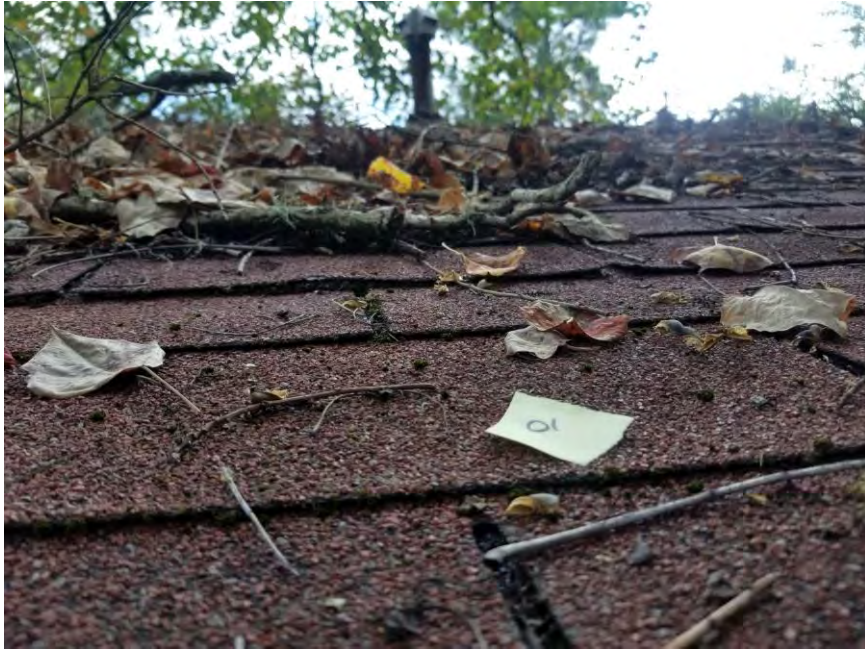
View of HA-01: Brown roof shingles and felt paper.
