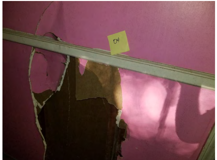
HA-04: White drywall with joint compound.
