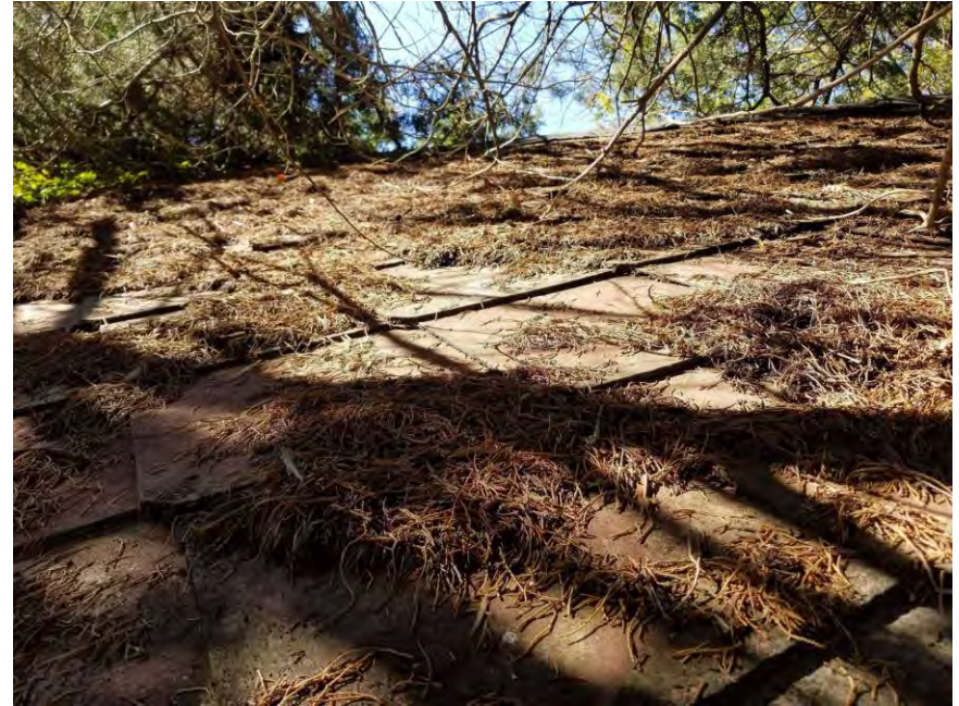
View of HA-06: Red-painted gray transite roof shingles with black tar.
