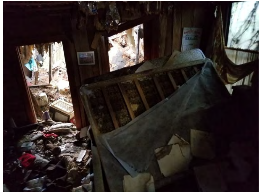
General view of interior.
