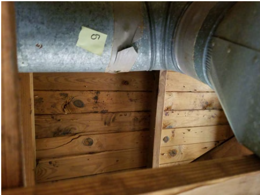
View of HA-07: White HVAC tape with tan mastic.
