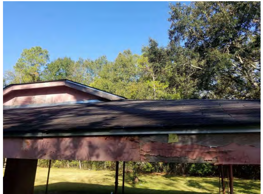
View of HA-08: Black roof shingles and felt paper.
