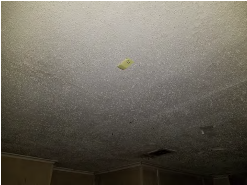
View of HA-01: White popcorn ceiling texture.
