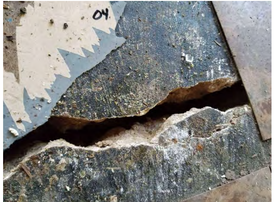
View of HA-04: Residual black mastic atop slab.
