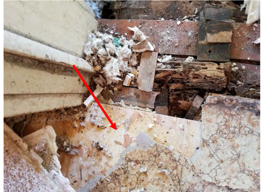
View of HA-07: Cream Sheet Flooring with Fiber Backing
