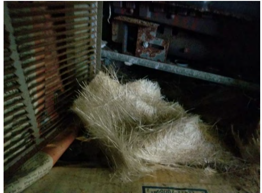
View of HA-08: White space heater insulation.
