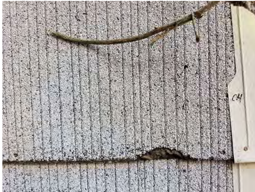
View of HA-04: Black Tar Shingle Siding
