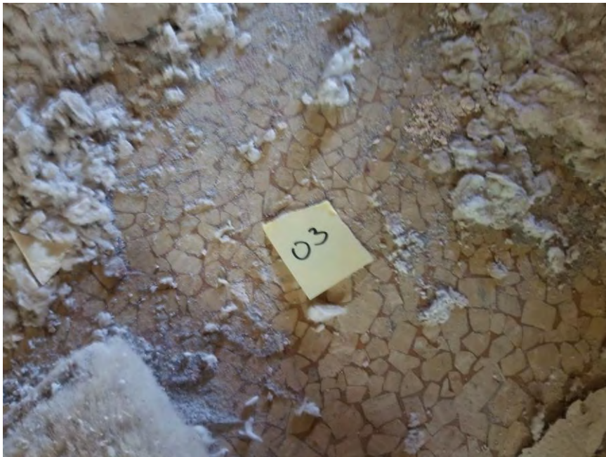
View of HA-03: Yellow sheet flooring with fiber backing.
