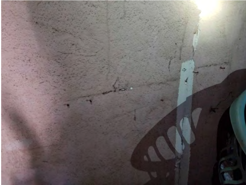
View of HA-01: White Wallboard with Joint Compound with Texture
