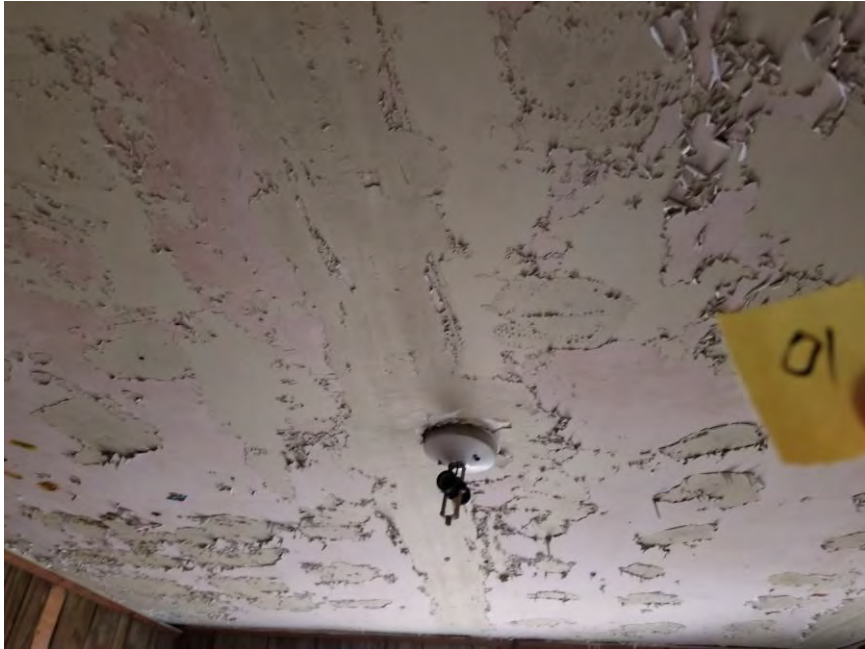
View of HA-01: White wallboard with joint compound and texture.
