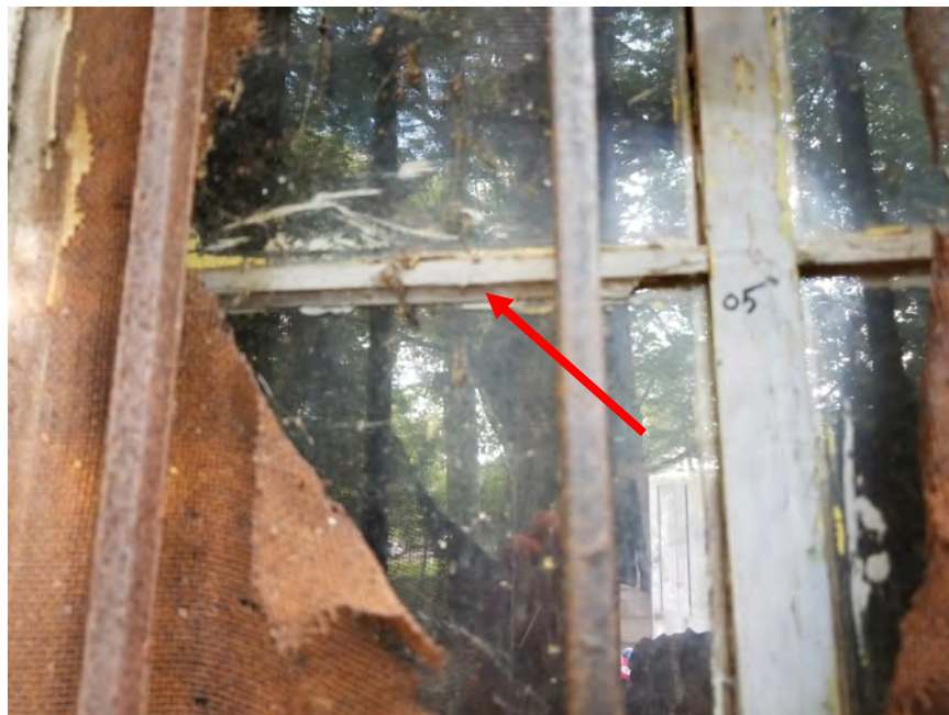
View of HA-05: Gray Window Glazing
