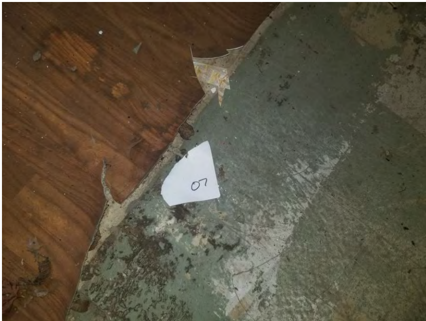
View of HA-07: Brown faux wood sheet flooring with fiber backing atop white faux ceramic tile sheet flooring with fiber backing.
