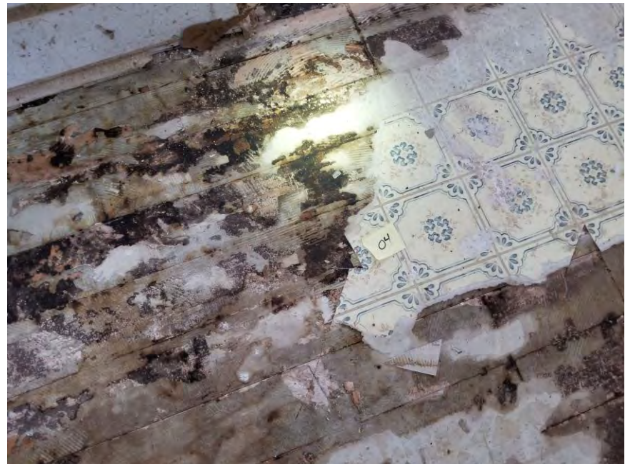
View of HA-04: Floral pattern sheet flooring with black mastic and fiber backing
