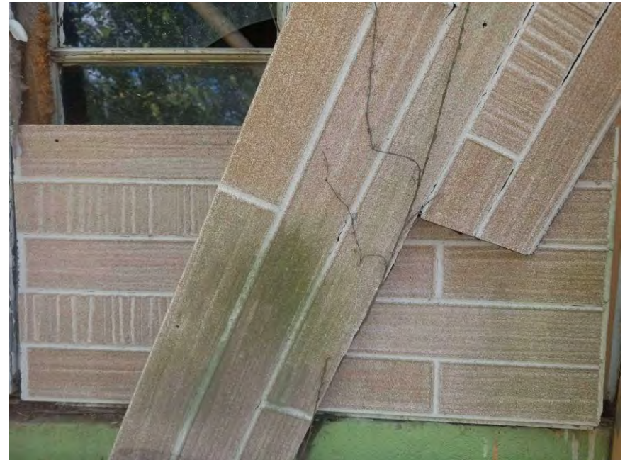
View of HA-06: Faux brick tar siding.
