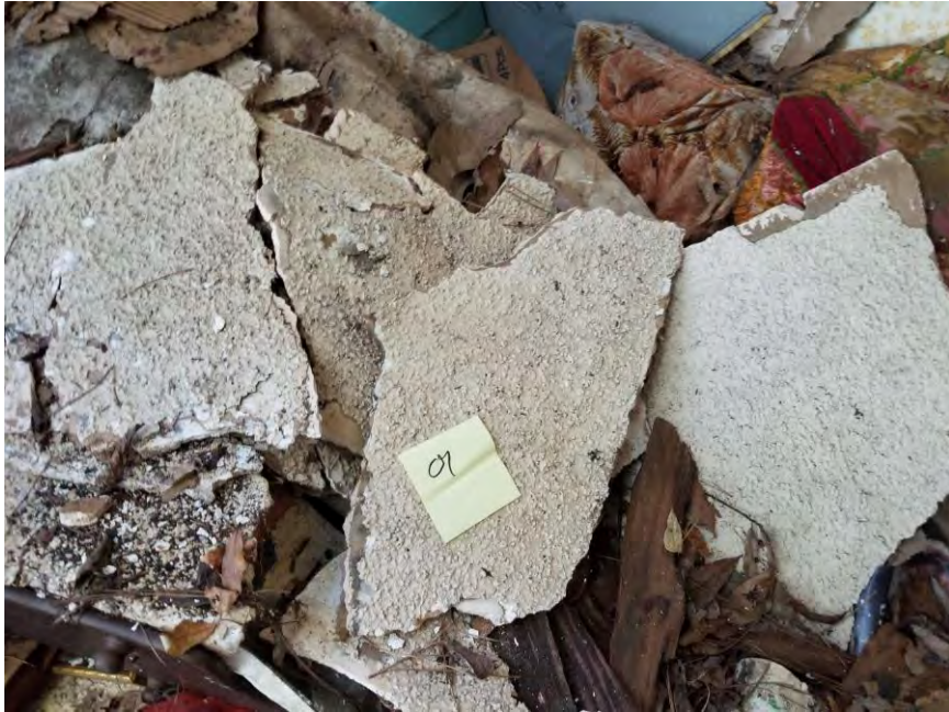
View of HA-01: White popcorn ceiling texture.
