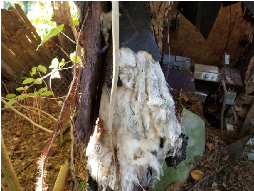
View of HA-07: White insulation.
