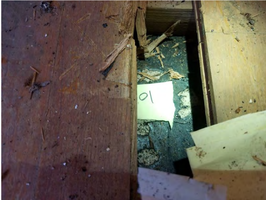
View of HA-01: Black sleeper tar underneath wooden floors.
