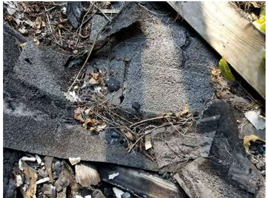
HA-04: Black Roof Shingles with Felt Paper
