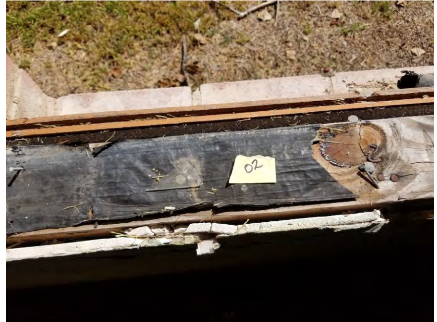
View of HA-02: Black vapor barrier.
