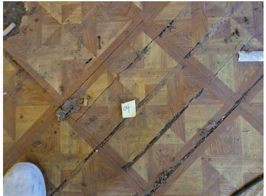
View of HA-04: Brown 12"x12" faux parkay self-stick floor tiles.
