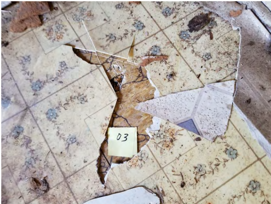
View of HA-03: Blue and white sheet flooring atop yellow sheet flooring atop brown 12"x12" floor tile with black mastic
