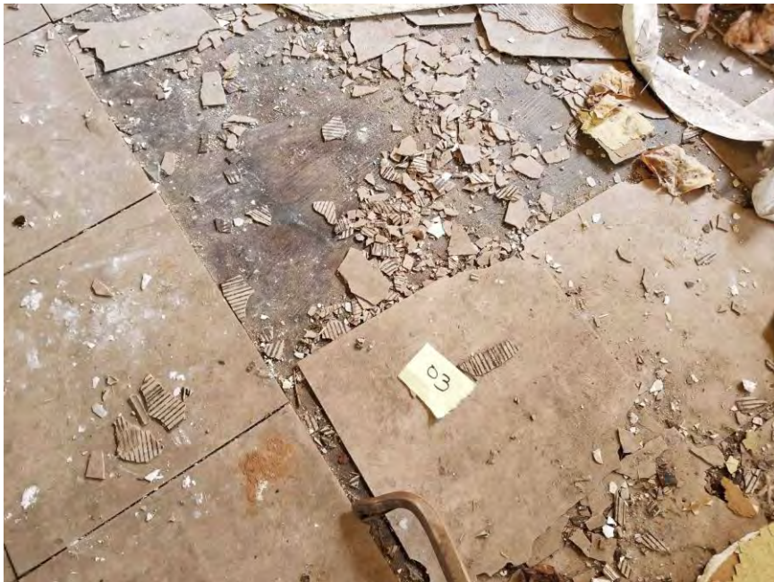
View of HA-03: Brown 9"x9" floor tile with black mastic.
