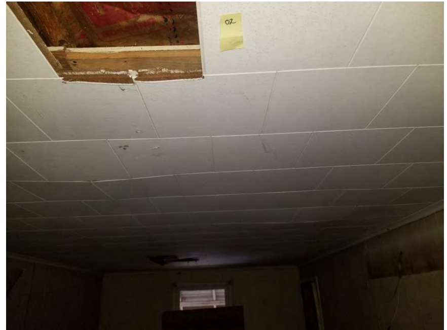
View of HA-02: White pinhole 1'x1' ceiling tile.
