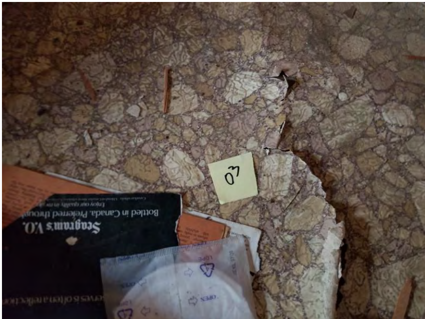
View of HA-03: Cream stone pattern sheet flooring.
