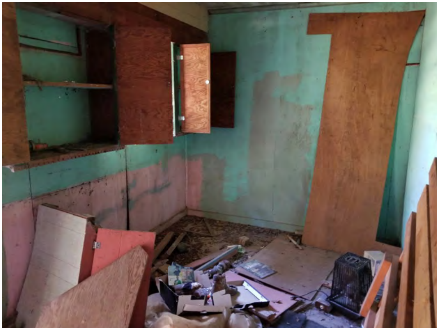
Another view of building interior
