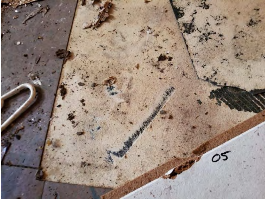
View of HA-05: Residual fiber backing atop residual black mastic.
