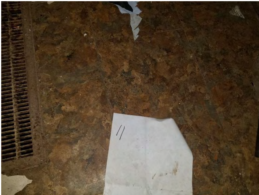
View of HA-11: Rust brown 12"x12" floor tile with black mastic.
