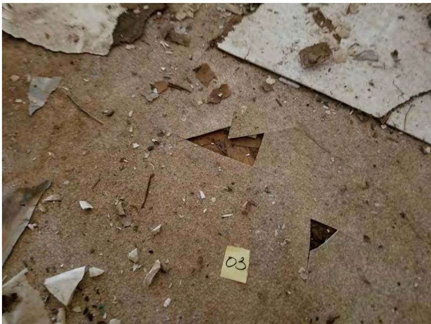
View of HA-03: Tan Pattern Sheet Flooring with Fiber Backing
