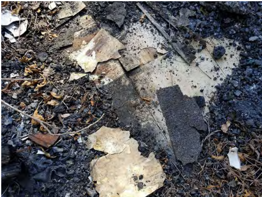
View of HA-03: 12"x12" Floor Tile with Black Mastic
