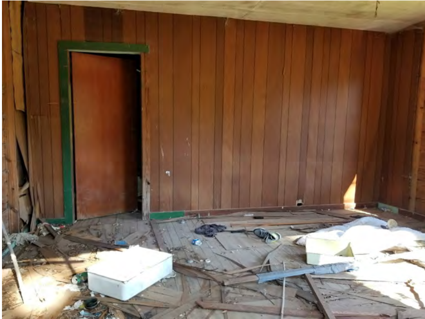
View of building interior.
