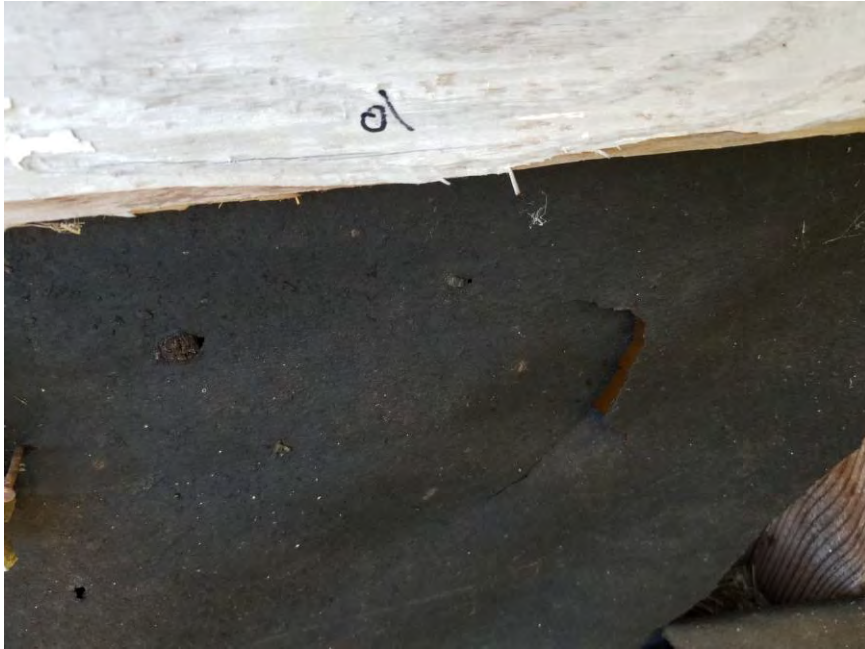
View of HA-01: Black vapor barrier.
