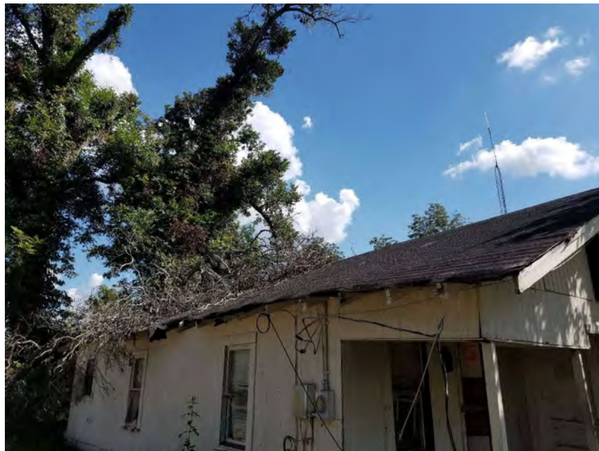
View of HA-06: Black Roof Shingles with Felt Paper
