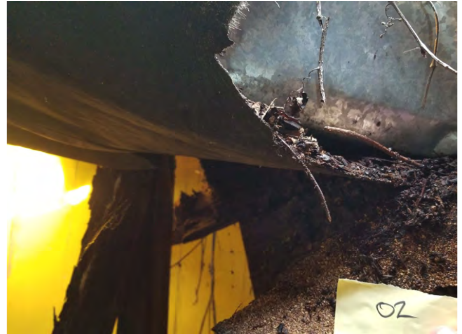
View of HA-02: Brown roof shingle with felt paper
