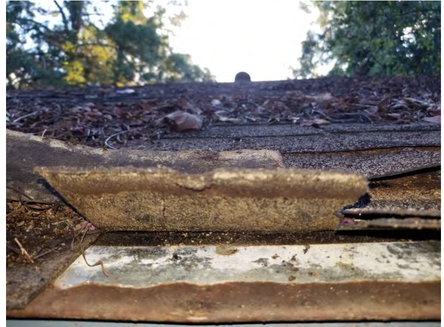
View of HA-14: Black roof shingle and black felt paper.
