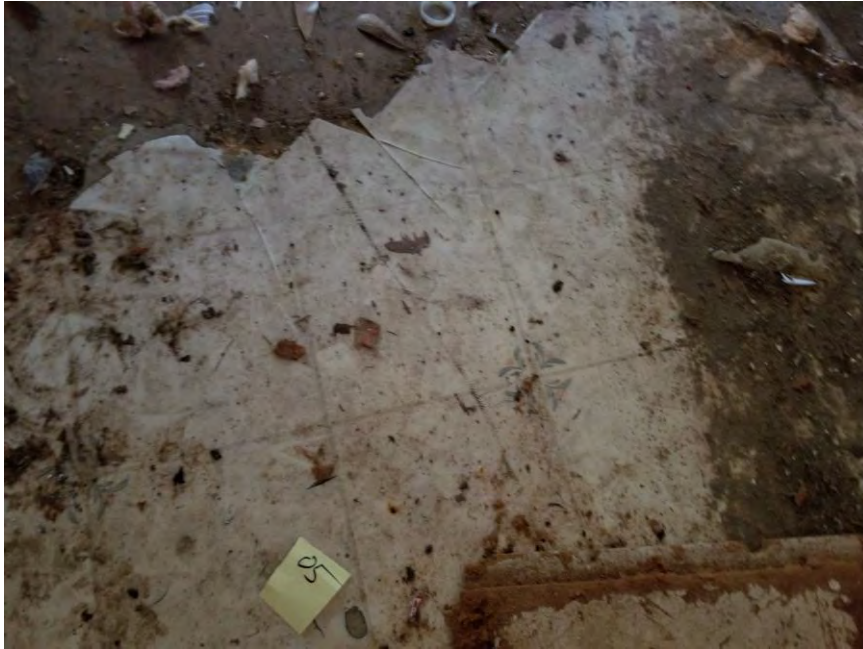
View of HA-05: White sheet flooring with 4"x4" pattern.
