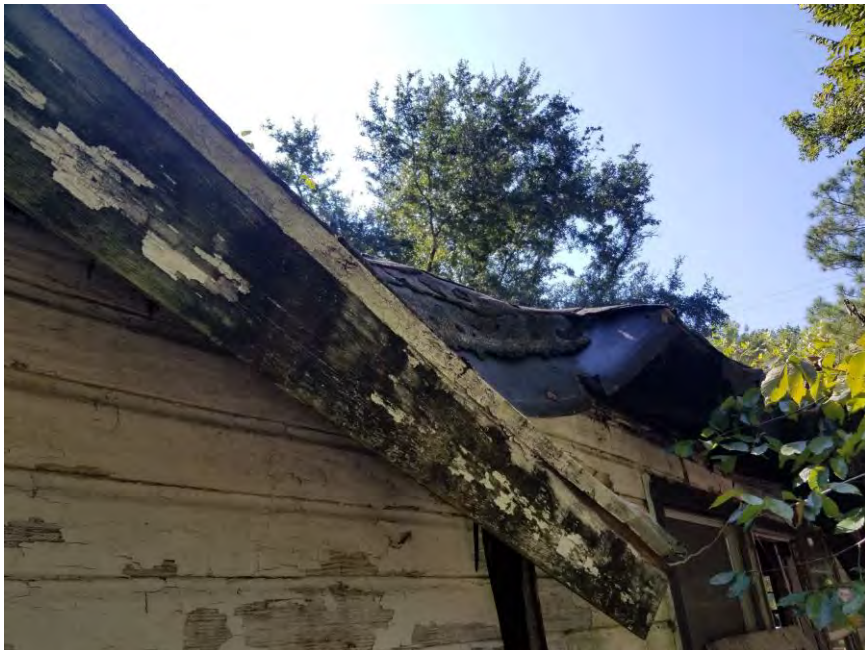
View of HA-12: Black roof shingles with felt paper.
