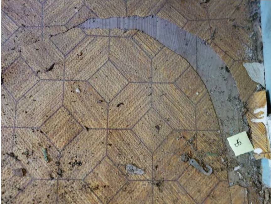
View of HA-05: Brown self-stick sheet flooring.
