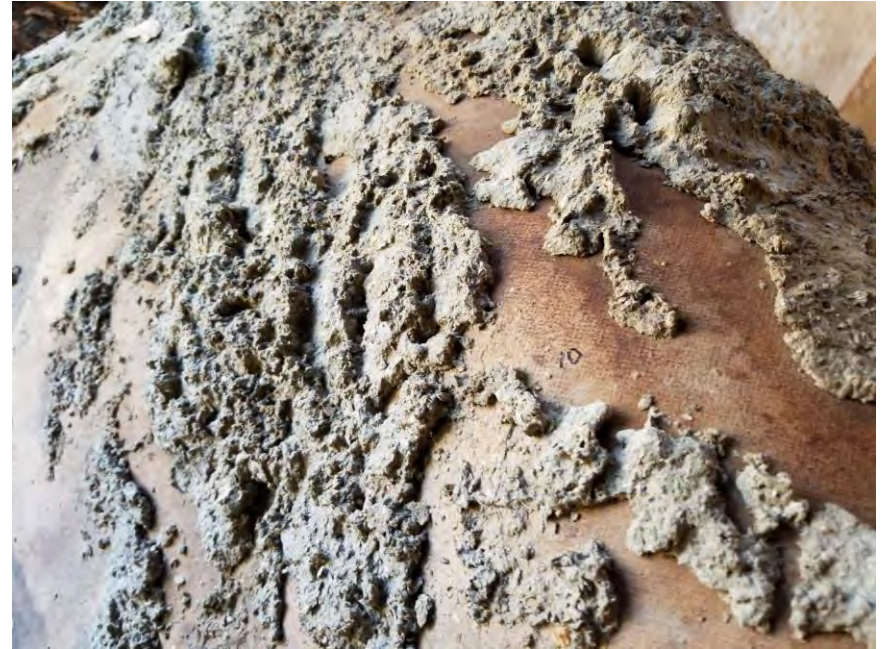
View of HA-10: Gray blown in insulation.
