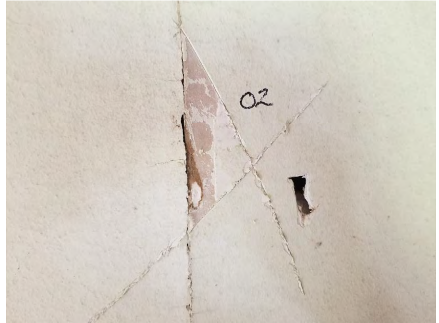
View of HA-02: White wallboard with joint compound and texture.
