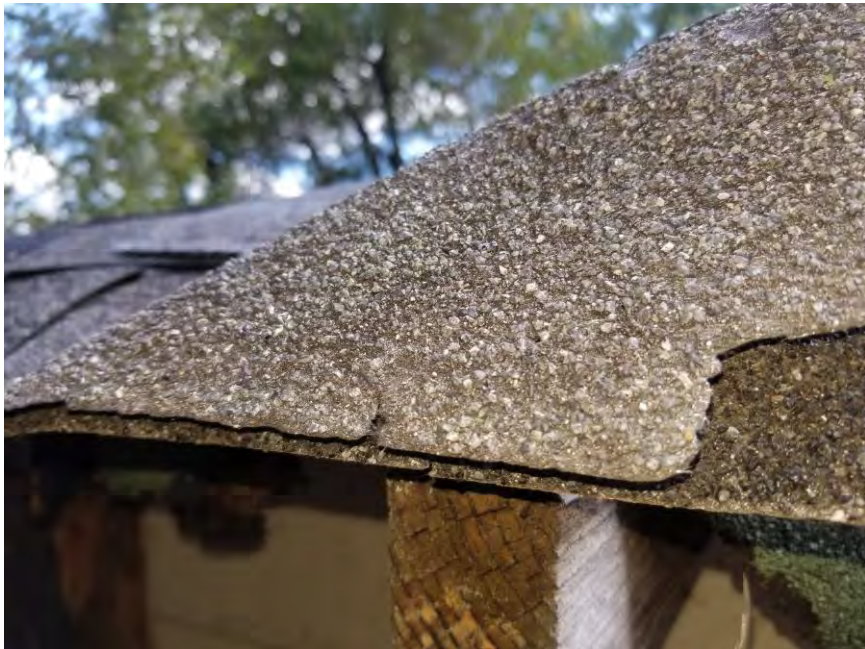
View of HA-05: Black and green roof shingle and felt paper.
