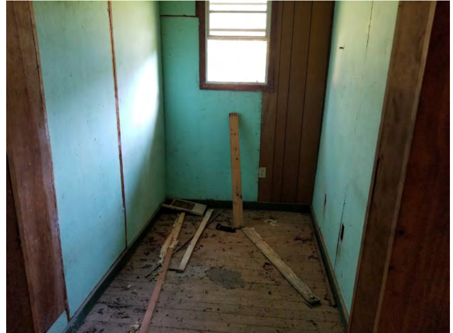
Another view of building interior.
