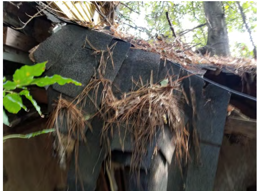
HA-05: Black roofing shingles with tar paper.
