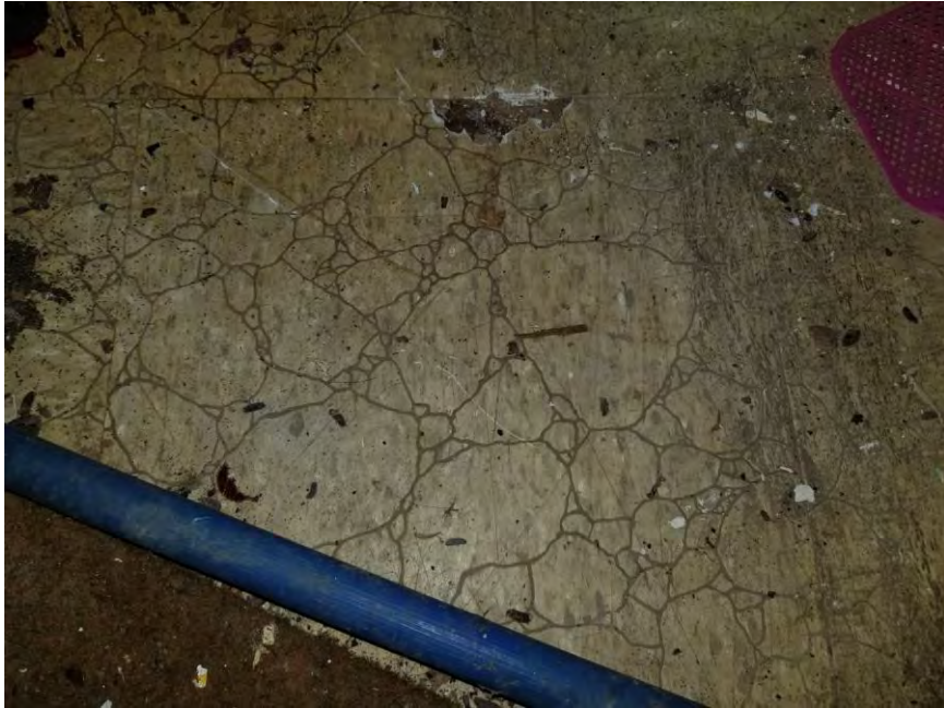
View of HA-01: Cream 12"x12" floor tile with yellow mastic.
