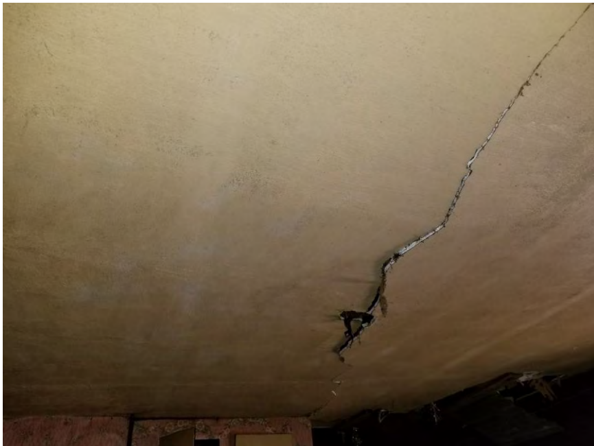
View of HA-03: White drywall and joint compound.
