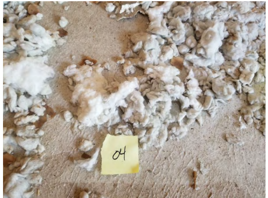
View of HA-04: Brown blown in insulation.
