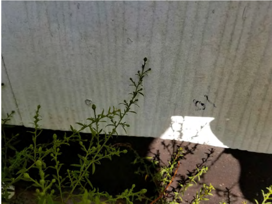
View of HA-01: White Transite Siding
