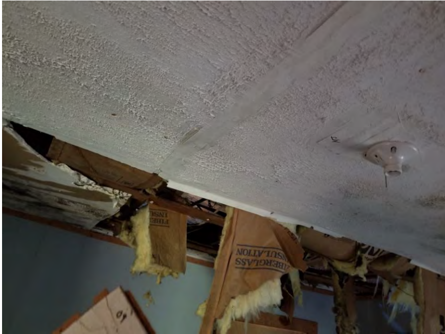
View of HA-09: White drywall with joint compound and texture.
