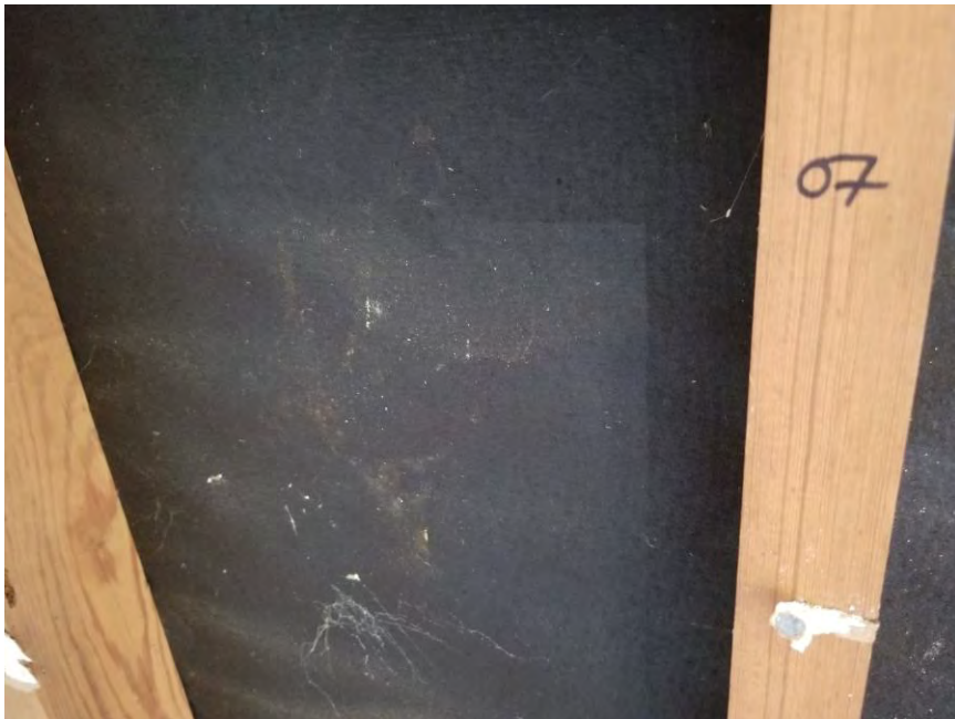
View of HA-07: Black vapor barrier.
