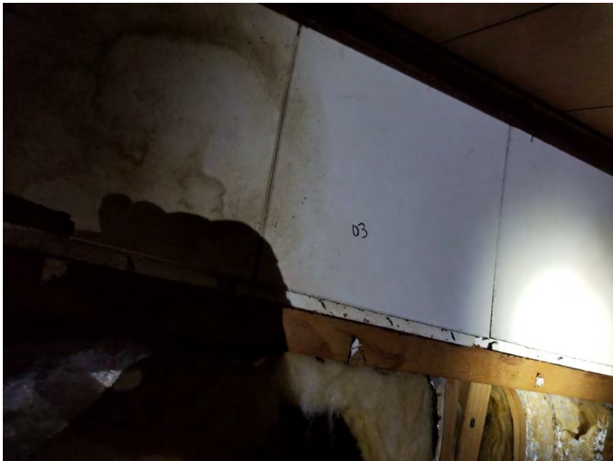
View of HA-03: White 1'x1' mechanically attached ceiling tiles.
