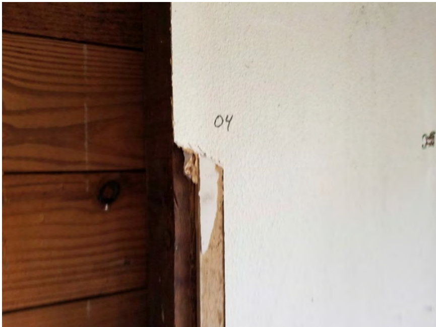
View of HA-04: White Wallboard with Joint Compound and Texture
