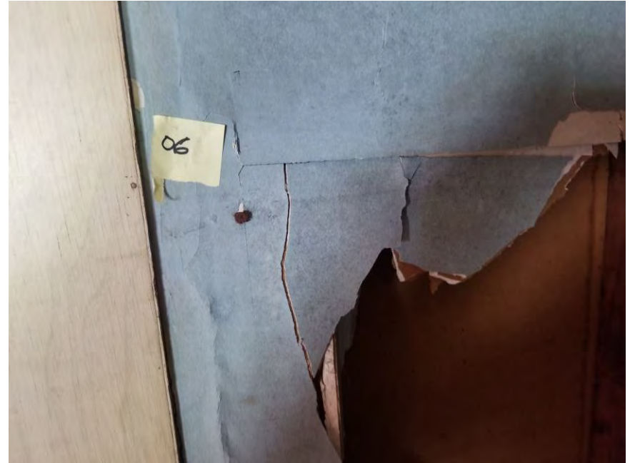
View of HA-06: White drywall with joint compound and texture.
