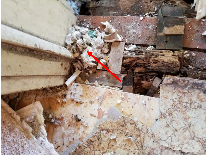
View of HA-06: White Blown-in Insulation
