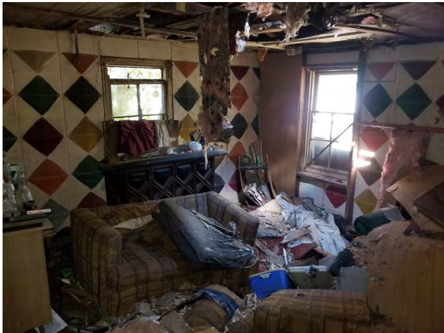
General view of the structure's interior.
