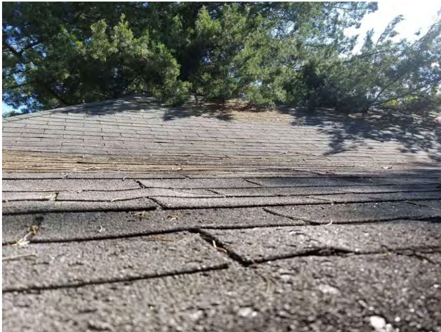
View of HA-07: Black roofing shingle and flashing.
