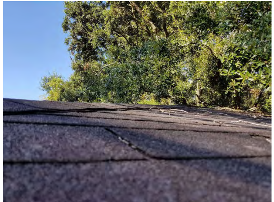
HA-01: Black Roof Shingles with Felt Paper
