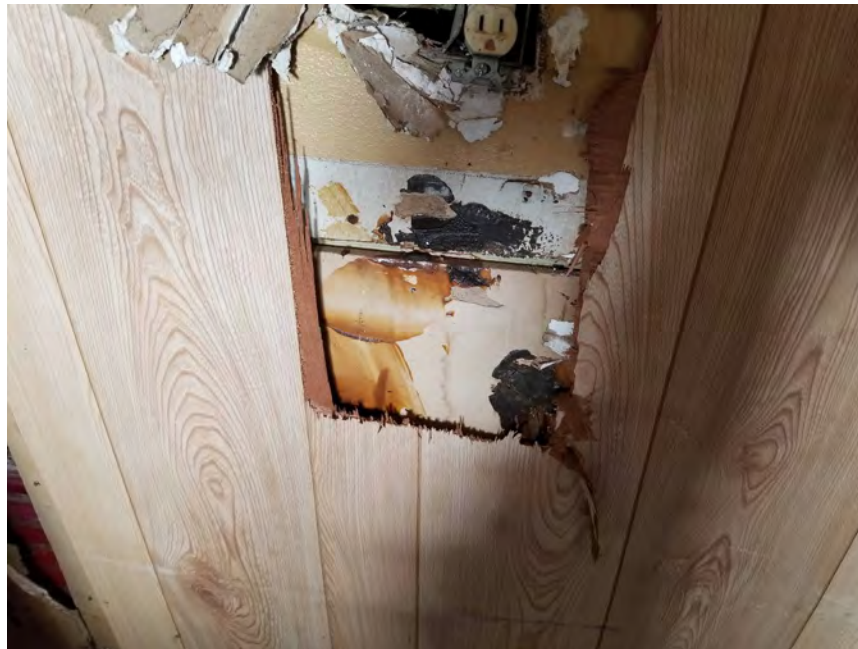
View of HA-08: Brown Wood Panel Mastic
