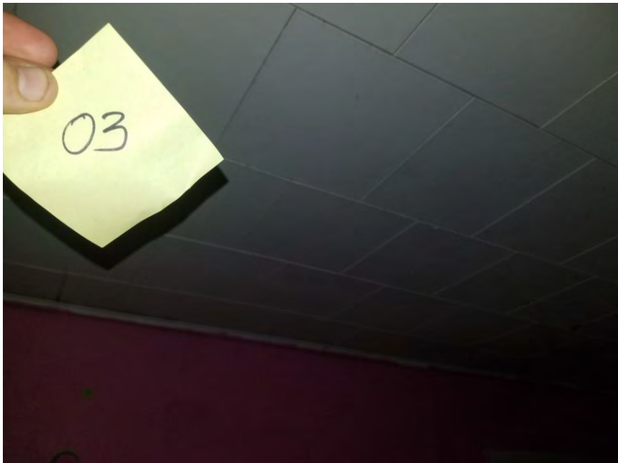
View of HA-03: Smooth white 1'x1' ceiling tile.
