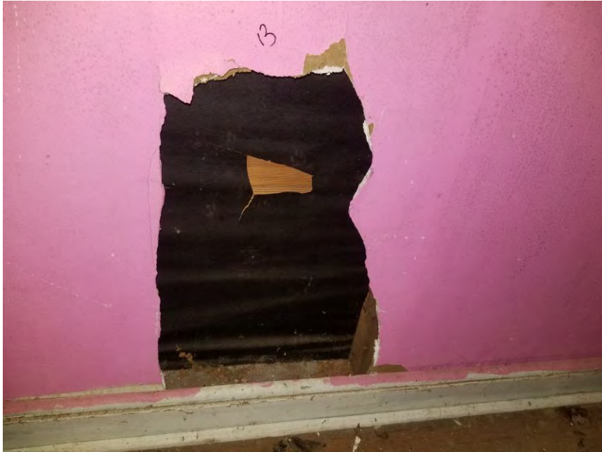
View of HA-13: Black vapor barrier.
