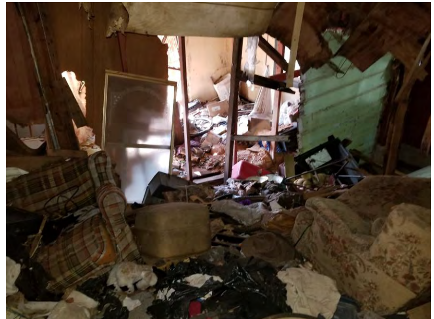
General view of the structure's interior.
