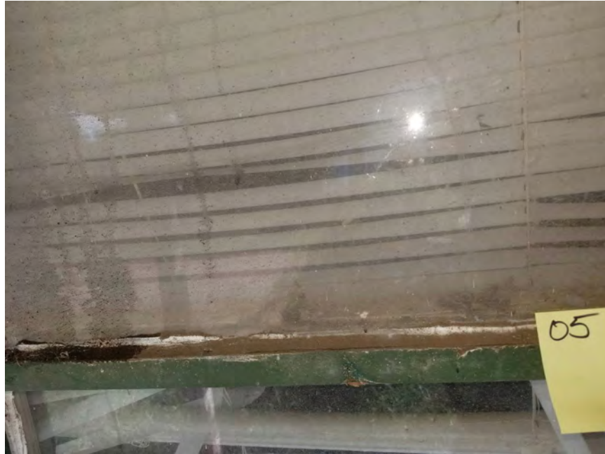
View of HA-05: White Window Caulking
