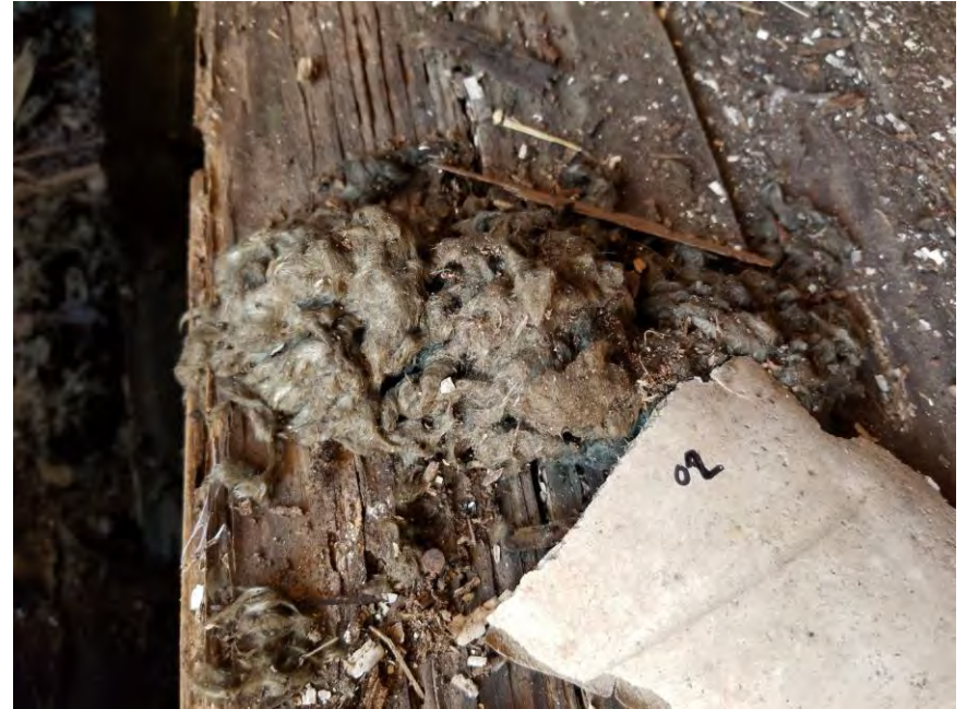
View of HA-02: Gray blown in insulation.
