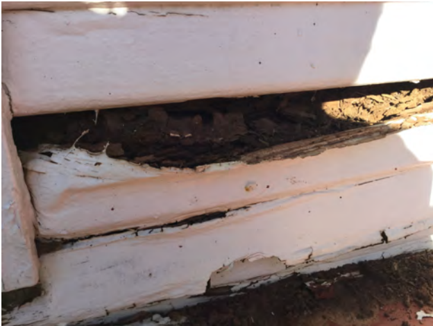
11/22/2017 1:53:57 PM Front porch. Right side at corner
