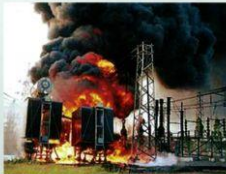
An example of a transformer fire
