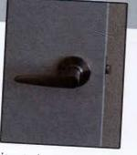
This exterior door hardware is compliant as it does not require pinching or twisting.
