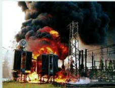
An example of a transformer fire
