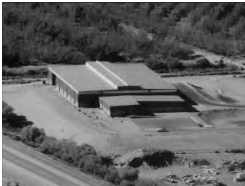
Aerial view of a totally enclosed transfer station.
