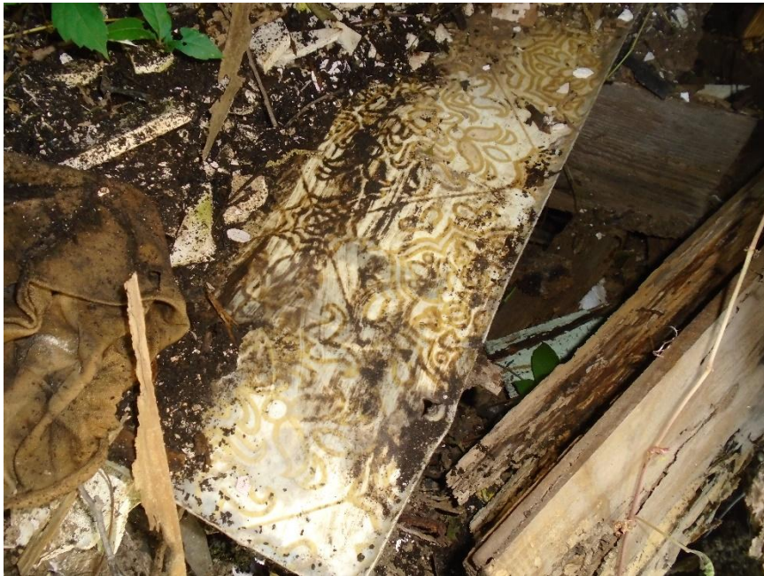
Photograph No. 3 View of HA-03: Cream Spanish Pattern Sheet Flooring.
