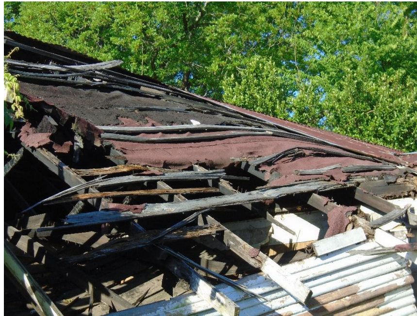
Photograph No. 9 View of HA-93: Red Roof Shingle
