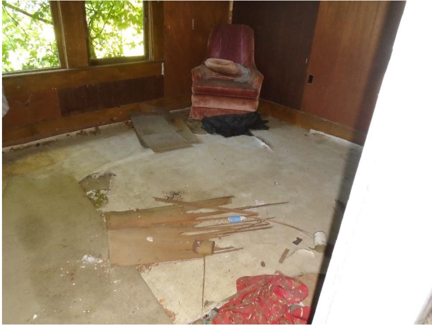
Photograph No. 4 View of HA-04: White 4" x 4" Square Pattern Sheet Flooring.
