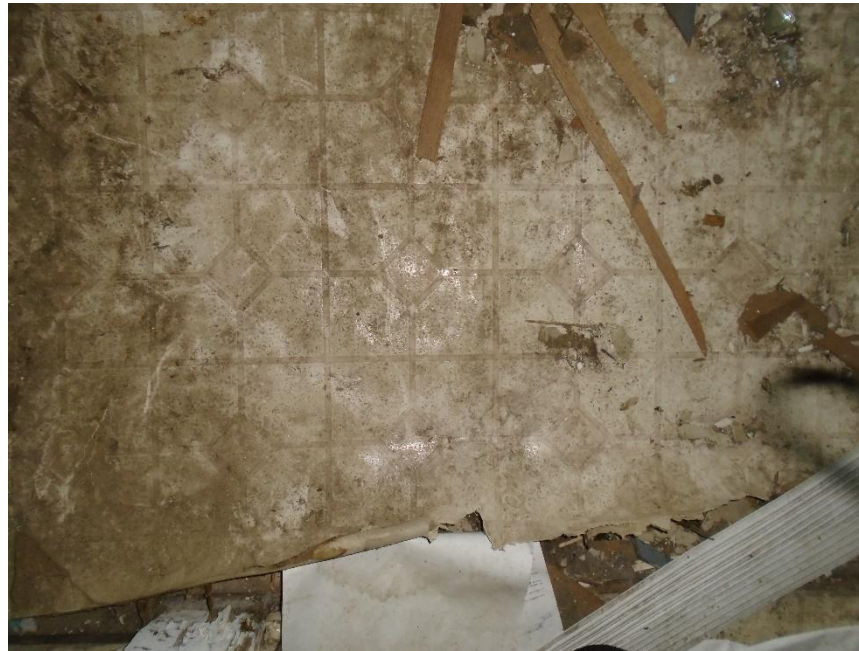
Photograph No. 3 View of HA-03: Tan Sheet Flooring with Brown Diamond Pattern.
