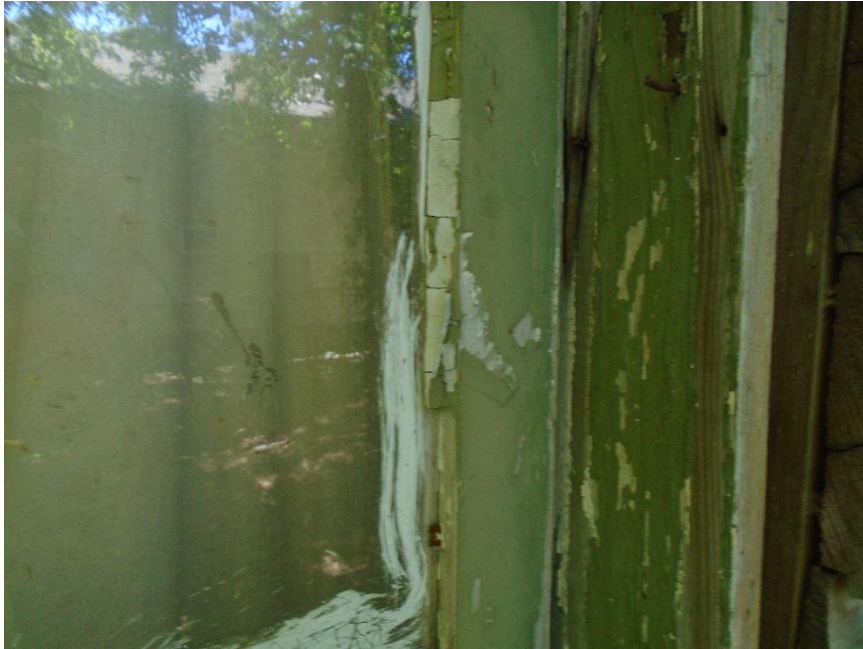
Photograph No. 1 View of HA-01: White Window Glazing
