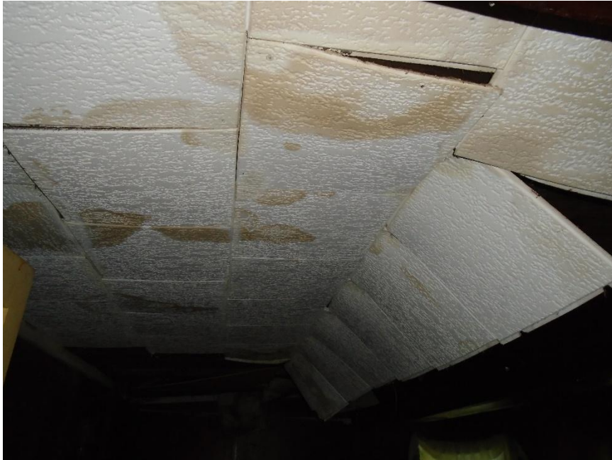
Photograph No. 5 View of HA-06: 1'x1' White Acoustical Tongue, and Groove Ceiling Tiles
