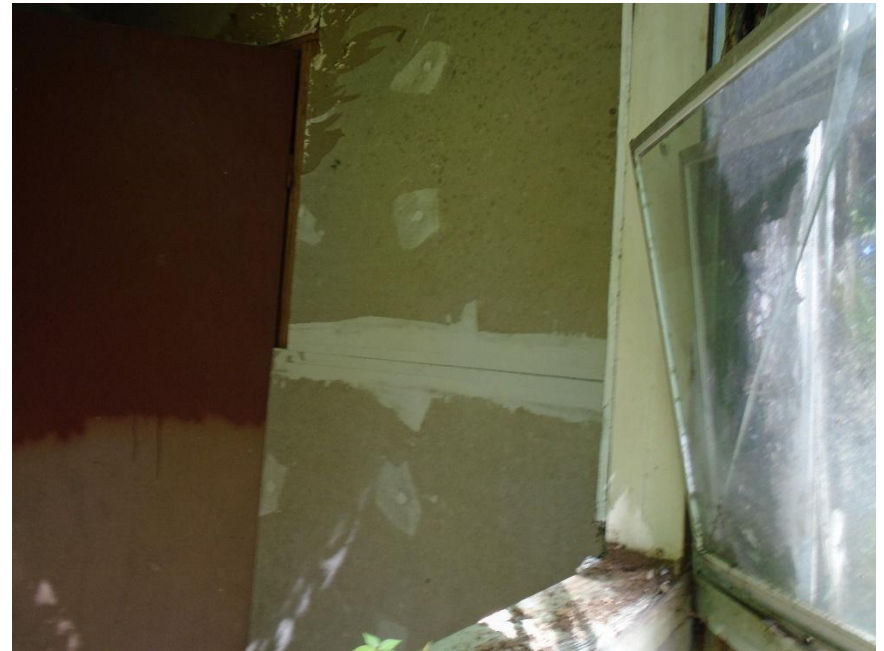
Photograph No. 4 View of HA-04: White Gypsum Drywall, Joint Compound, and Tape
