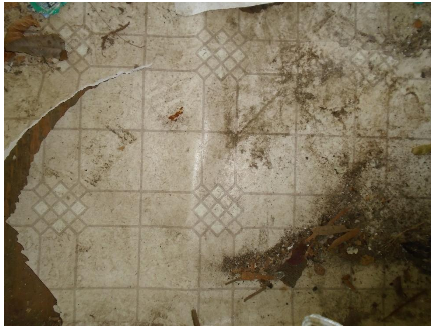
Photograph No. 6 View of HA-06: Tan Diamond Pattern Sheet Flooring.
