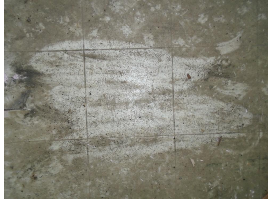
Photograph No. 8 View of HA-08: 6' x 6' Square Cream Pattern Sheet Flooring.
