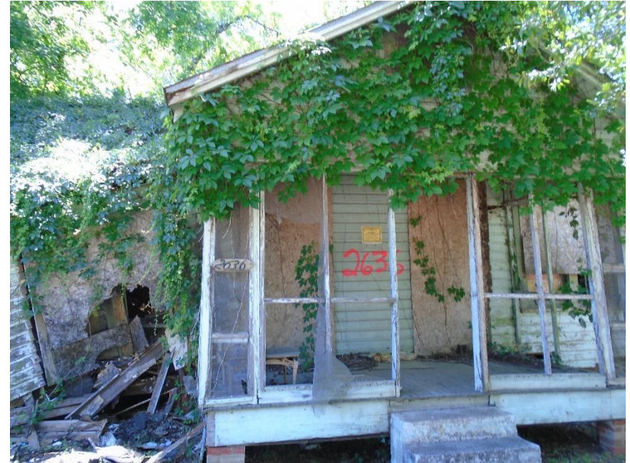
Photograph No. 2 View of HA-02 Black Asphalt Shingle.
