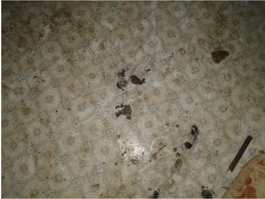
Photograph No. 1 View of HA-01: White Sheet Flooring with Blue Design.
