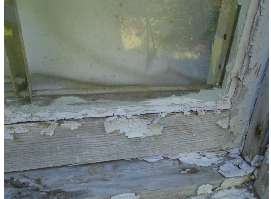
Photograph No. 6 View of HA-06: White Window Glazing.
