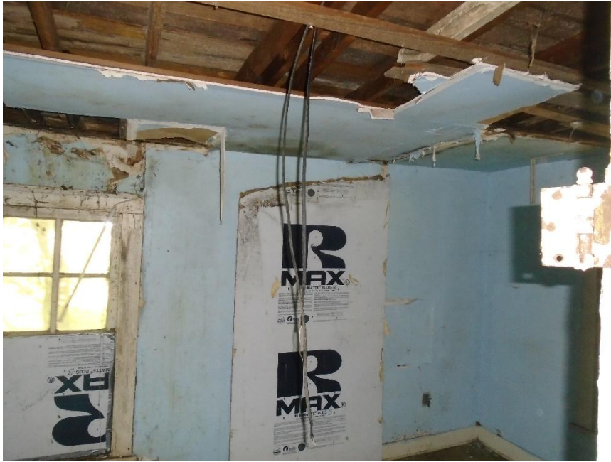
Photograph No. 5 View of HA-05: White Drywall Gypsum and Joint Compound.
