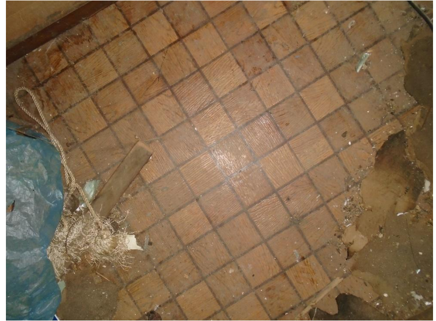
Photograph No. 2 View of HA-02: 2" x 2" Red Square Sheet Flooring.
