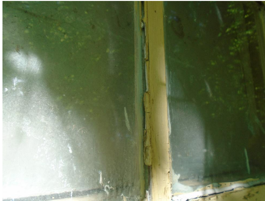
Photograph No. 7 View of HA-07: White Window Glazing.
