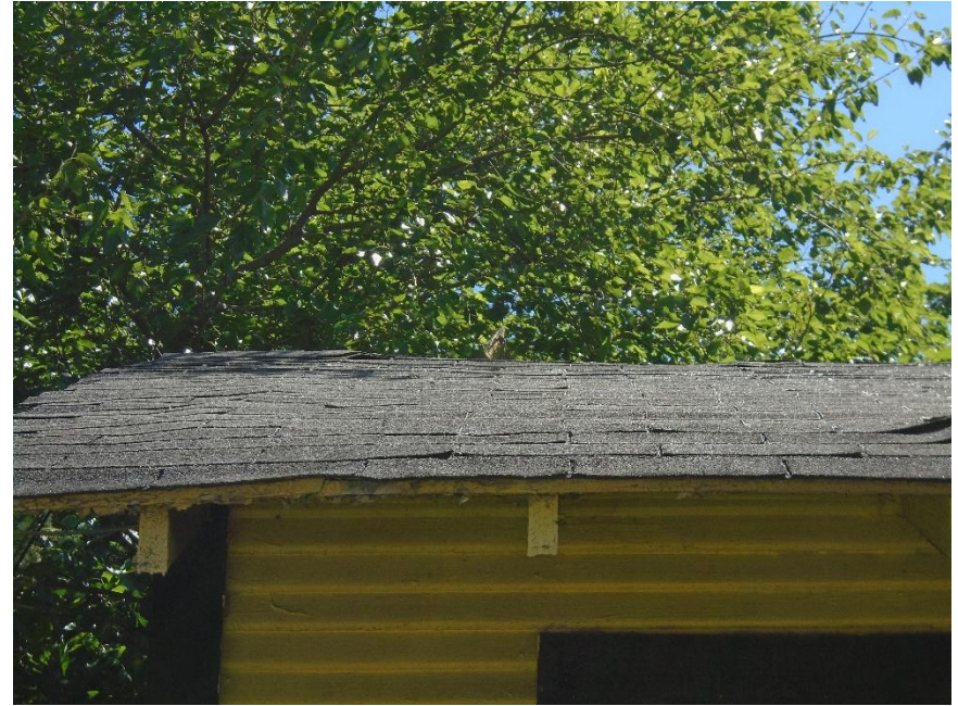
Photograph No. 6 View of HA-06: Black Asphalt Shingle.
