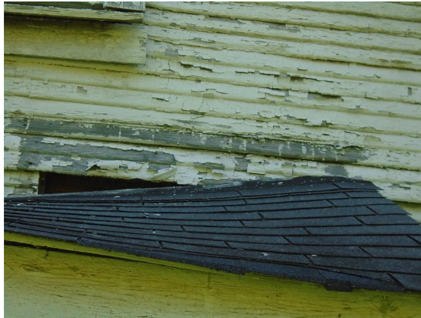
Photograph No. 7 View of HA-07: Black Roof Shingle
