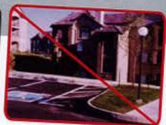
The lack of curb-cut makes this public space inaccessible.
