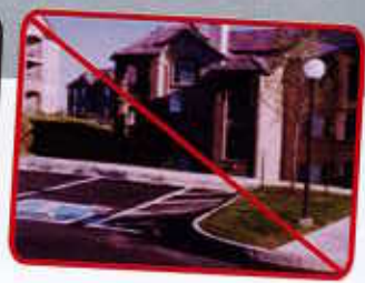
The lack of curb-cut makes this public space inaccessible.
