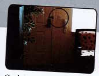
Outlet is correctly placed between 15" and 48".
