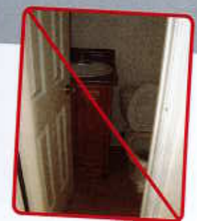
Lack of maneuvering space makes this room inaccessible.
